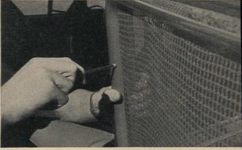
Screw the window molding back in place and trim off any protrudit edges of net. Replacing of molding automatically makes net snu
