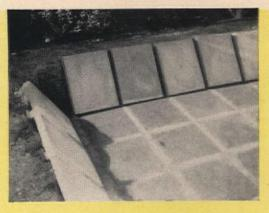
Lay bottom stones first and cement them, then lay side stones and cement. Use a little sand at bottom of hole to get stones firm and even.
