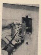
box and out this opening. Go outside house and hook both wires at one end of BX to coat-hanger wire; pull wires and cable connector into knockout in back of existing box. Attach connector firmly to box with lock nut. Reinstall inside receptacle being careful to attach both old and new white wires to lightcolored screws, and both old and new black wires to brass or dark-colored screws. Attach the new box to the other end of the
