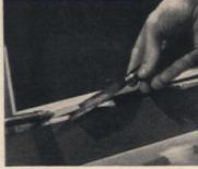
It is often difficult to remove the hard, dry putty around a broken window pane without chipping the window frame. An electric soldering iron softens the putty and makes it easy to lift out with a chisel.
