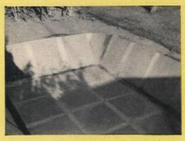
Make corners with 3" of gravel-mix cement and cover with smooth sand-mix. Shape with trowel or a tarpaper form. Pool can be emptied with garden hose siphon, or you can install a drain.
