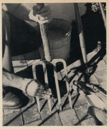
The first order of tool-care business is cleaning those implements that work the soil: forks, spades, shovels, hoes, cultivators, and such. Use steel-wool-and-soap cleansing pads to remove all dirt and rust, wash with clean water, dry completely, and then wipe thoroughly with heavy oil.
