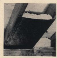
Staple batt or blanket insulation to the bottom edge of roof rafters. Space between insulation and roof boards provides room for air flow; helps keep roof boards dry, free from rot.
