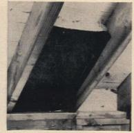
Staple insulation as shown. Lack of ventilation will rot roof boards. Black vapor barrier on insulation stops inside water vapor passage into wall, ceiling spaces.
