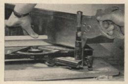
A good rule of thumb when joining moldings at corners: miter for outside corners, cope for inside. Set cove moldings, pattern up in the same position it goes onto wall, against the backguide of miter box. Trim off at a 45-degreeangle with miter saw.
