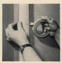
After the glue has set and dried, remove masking tape and sand with a fine grain sandpaper until splinter is invisible. This kind of blind nailing is especially good where the final job is to be clear-finished and where puttied nail holes would show through the clear finish. Keep glue clean or it will leave a dark line around the splinter outline.
