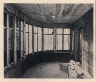
Opposite end of room clearly shows the rough state of the old greenhouse before new flooring, ceiling tile and furnishings were added. Cork tile was applied over the concrete floor to cut down reverberation from the brick wall and glass windows. Fifty feet of matchstick draperies hide old casement windows, yet admit plenty of light. Black mortar joints between bricks accentuate their rough texture. To increase their usefulness, radiators are masked with wooden cover that serves as table.
