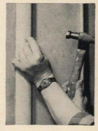
Next, drive the finishing nail into the wood behind the wood sliver. Use a nail-set to sink it beneath the surface of the molding and below the bottom of the sliver so that the sliver can fit back into place easily over the nail.
