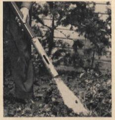
The Jet-Rod is a one-piece. lightweight flame gun for garden and other small-scale uses. It quickly kills weeds or unwanted grass, sterilizes surface soil, and melts ice or snow. It weighs less than 5 pounds and burns 30 minutes on one filling of 13/4 pints of kerosene. (The Geiger Company, North Wales, Pa.)
