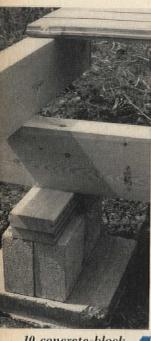
10 concrete-block piers on poured concrete footings are all the foundation required for this cabin. Over these are placed 4x8" girders which carry 4x8" floor joists.
