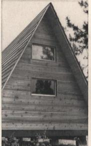
Rear of cabin is framed with 3x4" stock and covered with sheathing and cedar siding. Top window is for loft.
