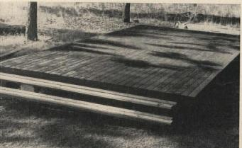
Floor for cabin is made out of 2x6" tongue-and-groove stock. Deck framework is covered with square edge 2x6s, set 1/4" apart.
