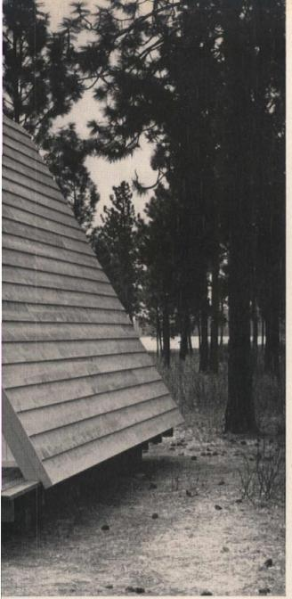
This cabin was built in 105 man hours or by two people working three full days. The materials, excluding plumbing and wiring, cost under \$1000 in the State of Washington.
