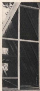
Front of cabin framing accommodates door and fixed or movable sashes. Siding used is 34" tongue and groove.
