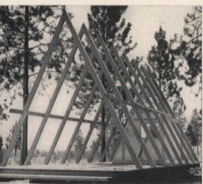
Frames are set in place, braced, and nailed into decking or bolted to the projecting ends of the floor joists.
