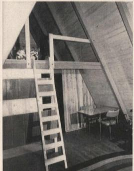
Enclosed area of cabin measures 16x22'. Because of A-frame construction, dimensions can easily be increased or decreased.
