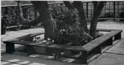
Bench around a tree is made from 2x2s of graduated lengths. Ends are butted to form a square. An air space of ½-½" should be left between seat members for drainage. Supports are 2x12s resting on ground with a cleat at the top. Supports at the corners are set at 45° angle. Seat members are nailed to cleats—outer members should extend 1" beyond cleats but members at inner edges should be flush.
