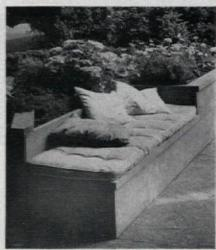
Island planter bench is basically a 90° triangle. Sides of bench (including back and side of seat) are 2x12s. Structure is supported at three corners by 2x4" posts. Seat is of 2x8s and extends 1" at the edges. Sides of planter are nailed to posts; topped with 2x8" cap rail.
