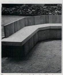
Boomerang bench has boxlike frame of 1x4s, lateral cleats of 2x4s at angle turns. Back and kickboard are vertical 2x6s nailed to frame, starting 2" above ground. Seat members are 2x4s extending beyond frame at ends. Boards of 1x4s cover edge of seat and kickboard.
