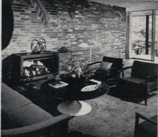
prick wall behind the fireplace separates the living-dining room and kitchen. Fireplace was custom-designed by Mr. Peiffer, is wall-hung, has double layers of steel with insulation between. Flue goes through kitchen cupboards. Deck is visible outside living room. Openness of rooms inside is ideal for letting tree tops become part of decor. The interior woodwork is hand-rubbed, oiled walnut, with concealed hardware.
