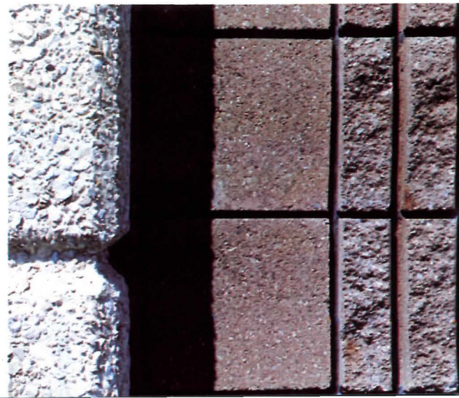
Detail of the exterior concrete masonry facade.
