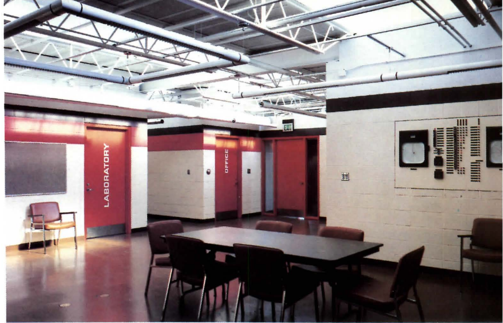
An interior scene with exposed concrete masonry walls used for heat storage and the clerestories above.
