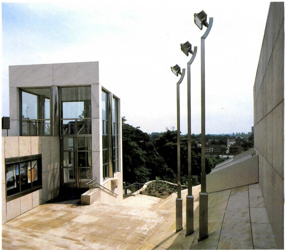
Top, site plan with serpentine, walled path. Above, the entrance pavilion. Across page, acropolis-like view from below.
