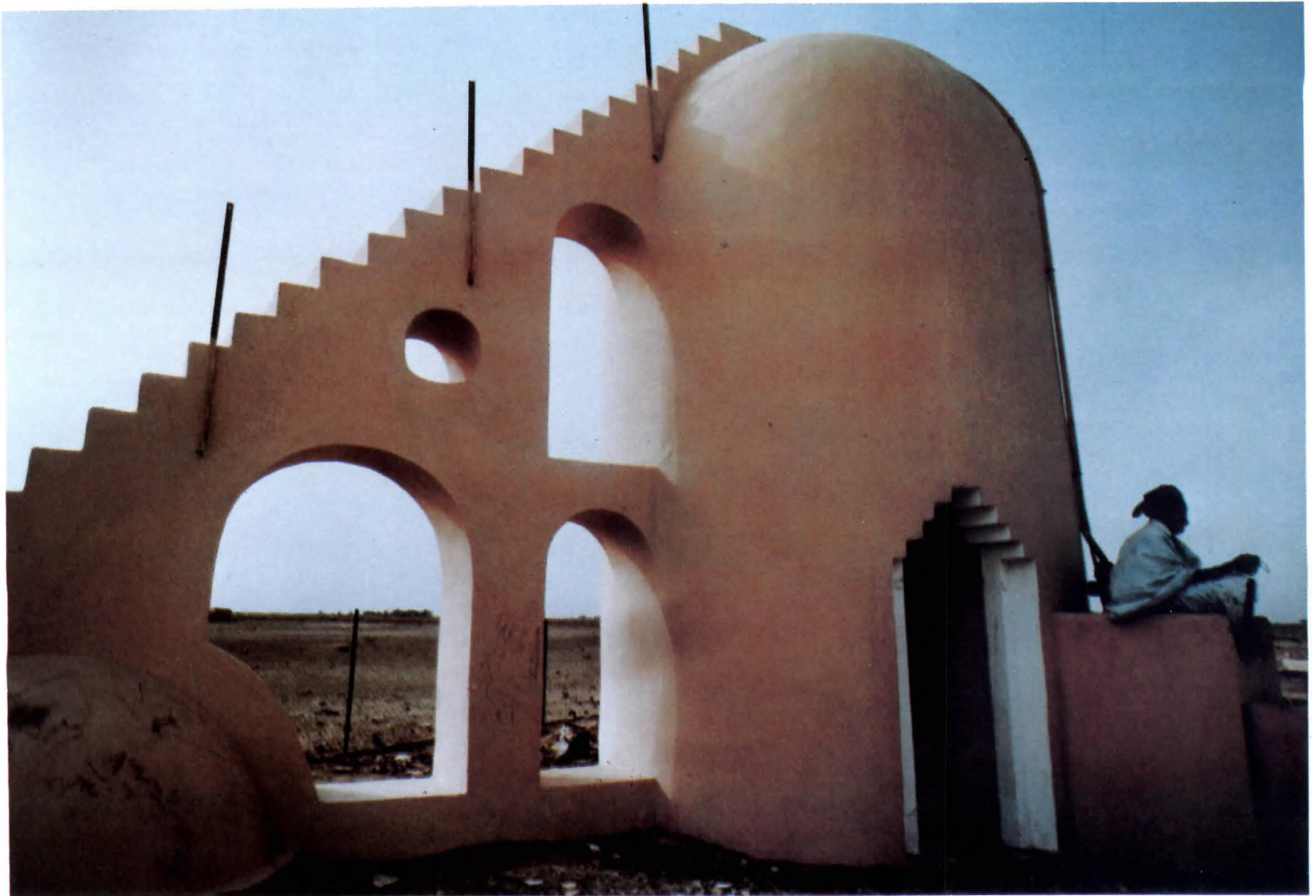
Project's roofline of low vaults and domes, left above, contrasts with traditional squatter housing, below. Above, water tank.
