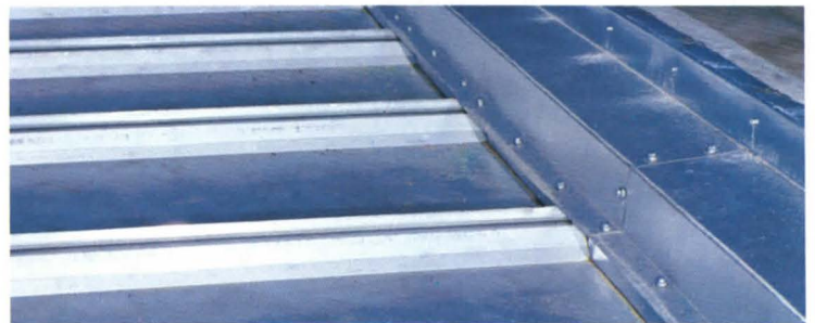
Roof-wall interface details for parapet wall.
