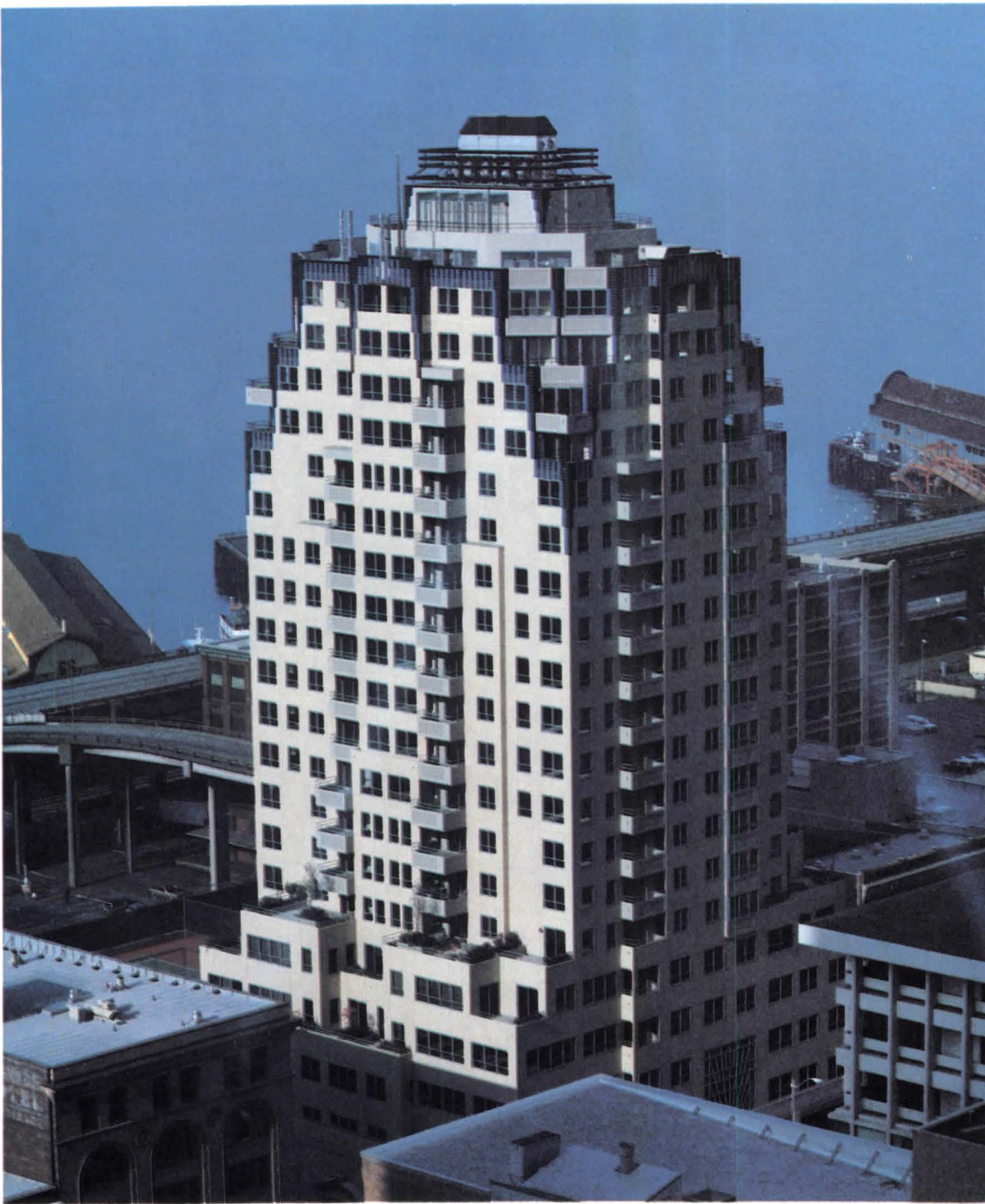
Multicolored zigzagging crown creates balconies and visual interest, across page. In a waterfront district of historic buildings, Watermark's southeast elevation includes preserved facade and entrance of a 1915 structure, below. Main entry is left, below.
