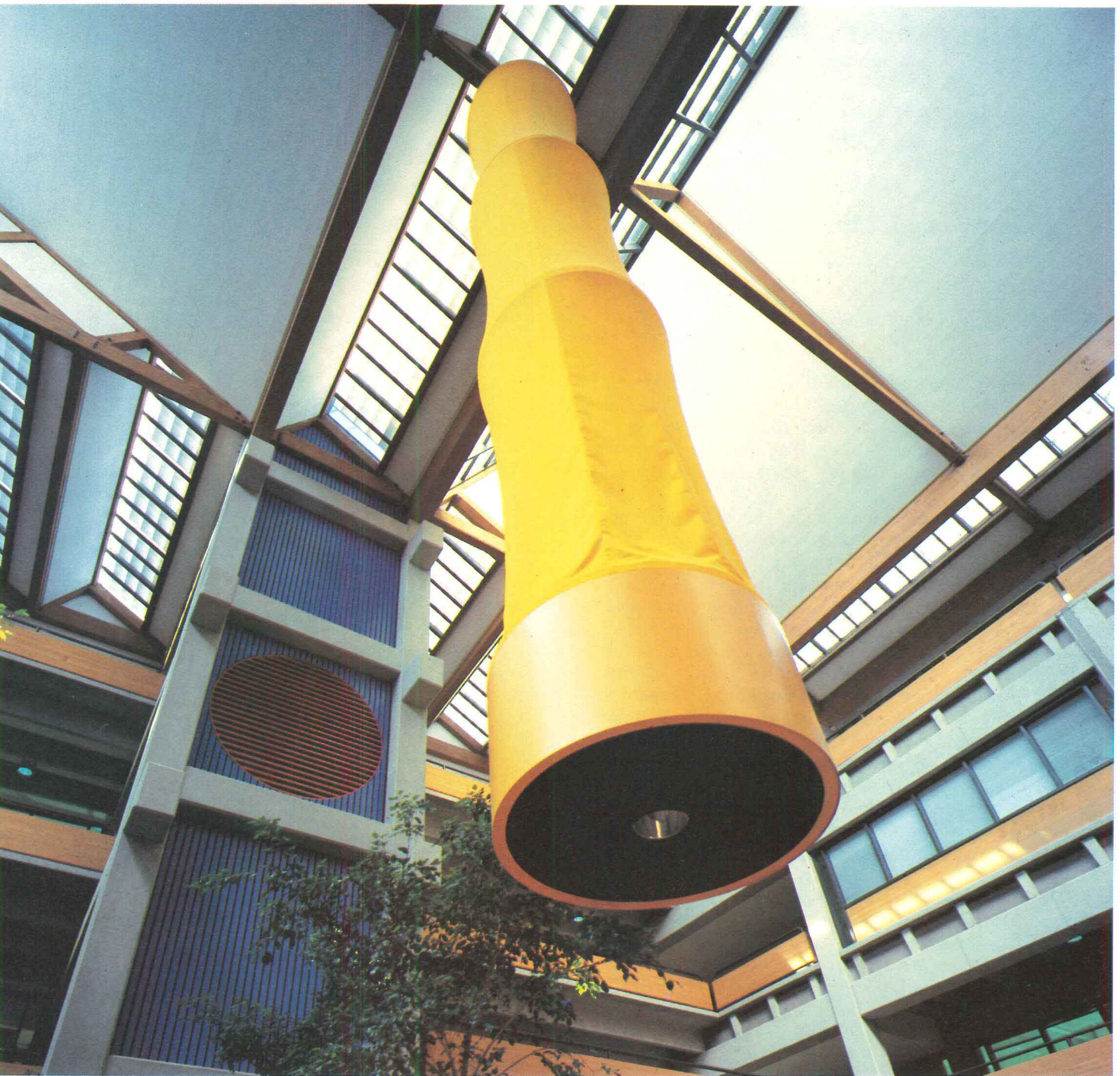
Left, condominiums (under construction) and gabled town houses; near left, apartments, all components of Somerset Parkside. Above, colors enliven the Bateson building atrium.
