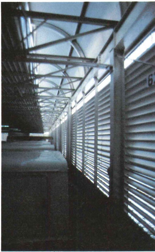
Mirror glass sheathes most of Viacom, except for garage, left, where open louvers permit natural ventilation. Roof monitors, section, bring light to interior, bottom right.
