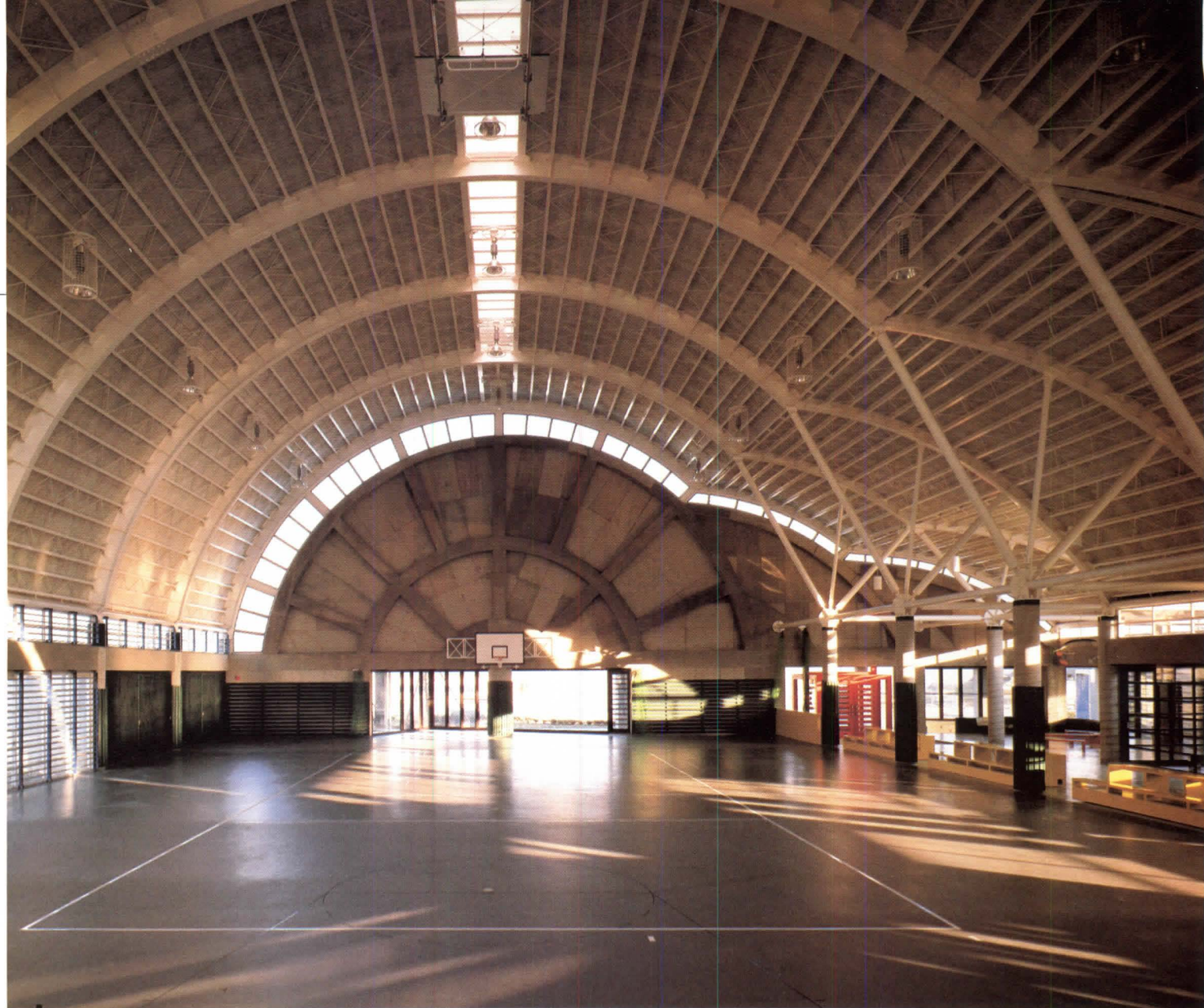
Three parallel vaults of different sizes create a cloud image, with portico, left below, masking the base. Glazing traces the exposed structure, emphasizing the shape of vaults while providing daylight.
