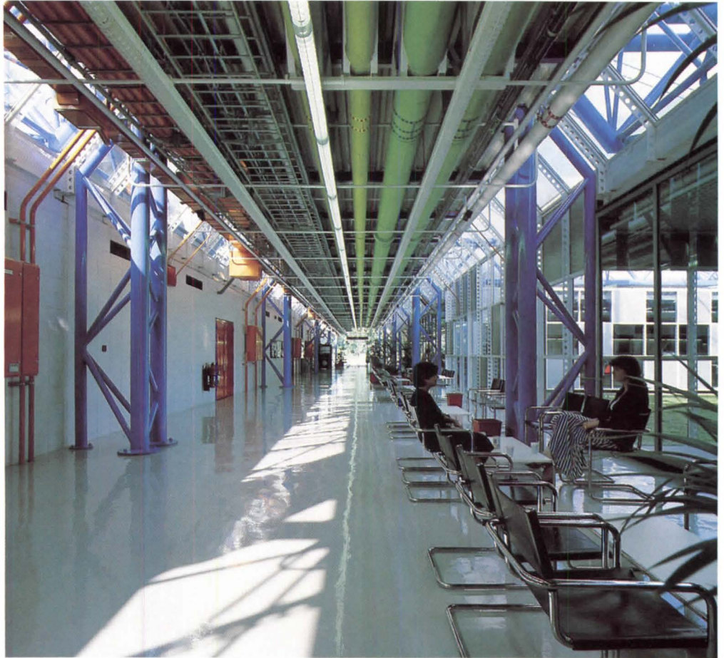
Sequence of giant blue H-frames across a green Welsh field, top. Rear entrance is across page, interior spine with continuous roof light is above.
