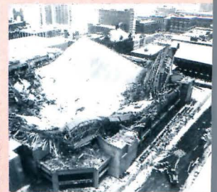
Shear forces generated by seismic ground motion, wind, and snow load are especially devastating to rigid structures. Because wood-frame design is more elastic, it dampens these stresses for higher margins of survivability.
