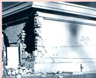
Shear forces generated by seismic ground motion, wind, and snow load are especially devastating to rigid structures. Because wood-frame design is more elastic, it dampens these stresses for higher margins of survivability.
