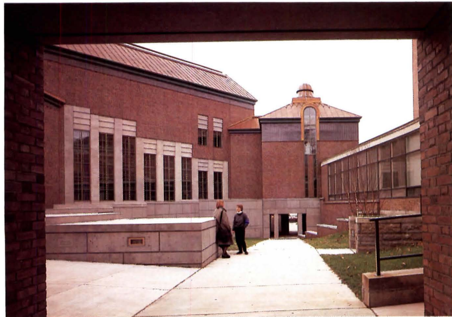
Top, the Hood's concrete and copper entry gate from the north, between Hopkins Center and Wilson Hall; above, view of the courtyard framed by the gate, with far portal leading to second courtyard. Across page, reception area near entry vestibule.
