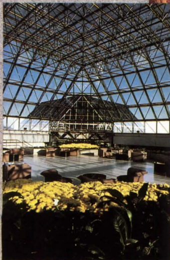
Atrium center of the Intelsat building in Washington, D.C.
