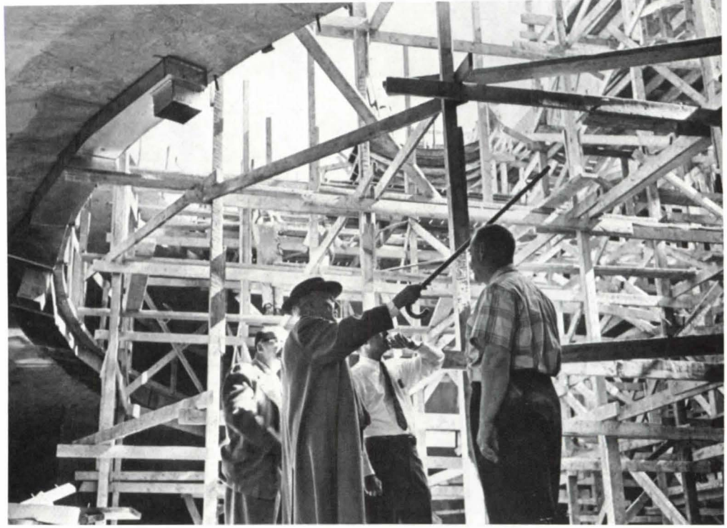
Wright inspects museum under construction.
