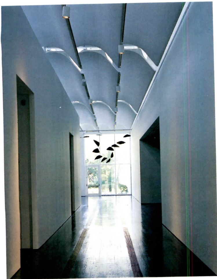
Left, first-floor corridor, typical of galleries, with stark white walls, air supply grilles in floor, and lighting tracks at the lower edge of diffusers. Right, view from sculpture gallery into unenclosed, shaded courtyard, to another gallery.
