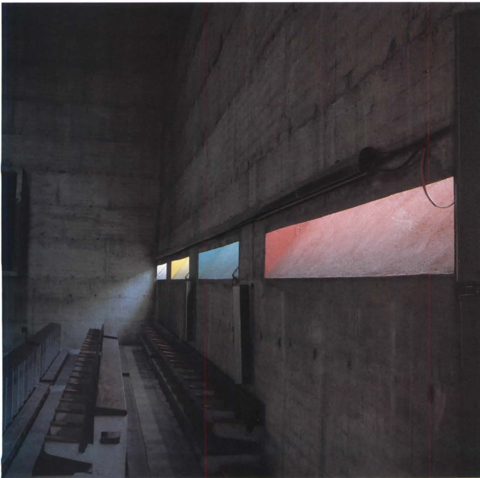
Above, splashes of sky in the blue chapel of Ronchamp. Left, at Le Corbusier's Monastery of La Tourette at Eveux-sur-l'Arbresle, angled light canals are sliced into the deep wall. Right, whitewash on plastic volumes in Ostuni, Italy.
