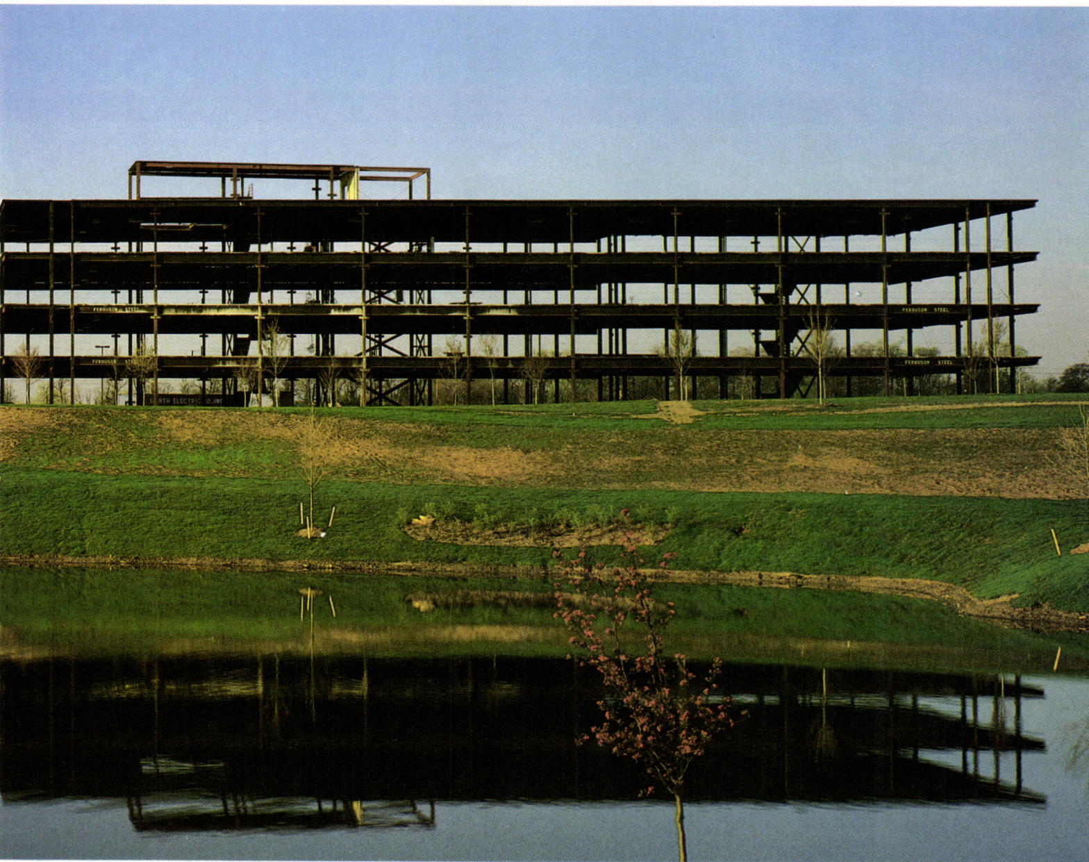
The Woodfield at The Crossing office complex in Indianapolis used 216 tons of Vulcraft joists and 169,000 sq. ft. of Vulcraft steel deck.
