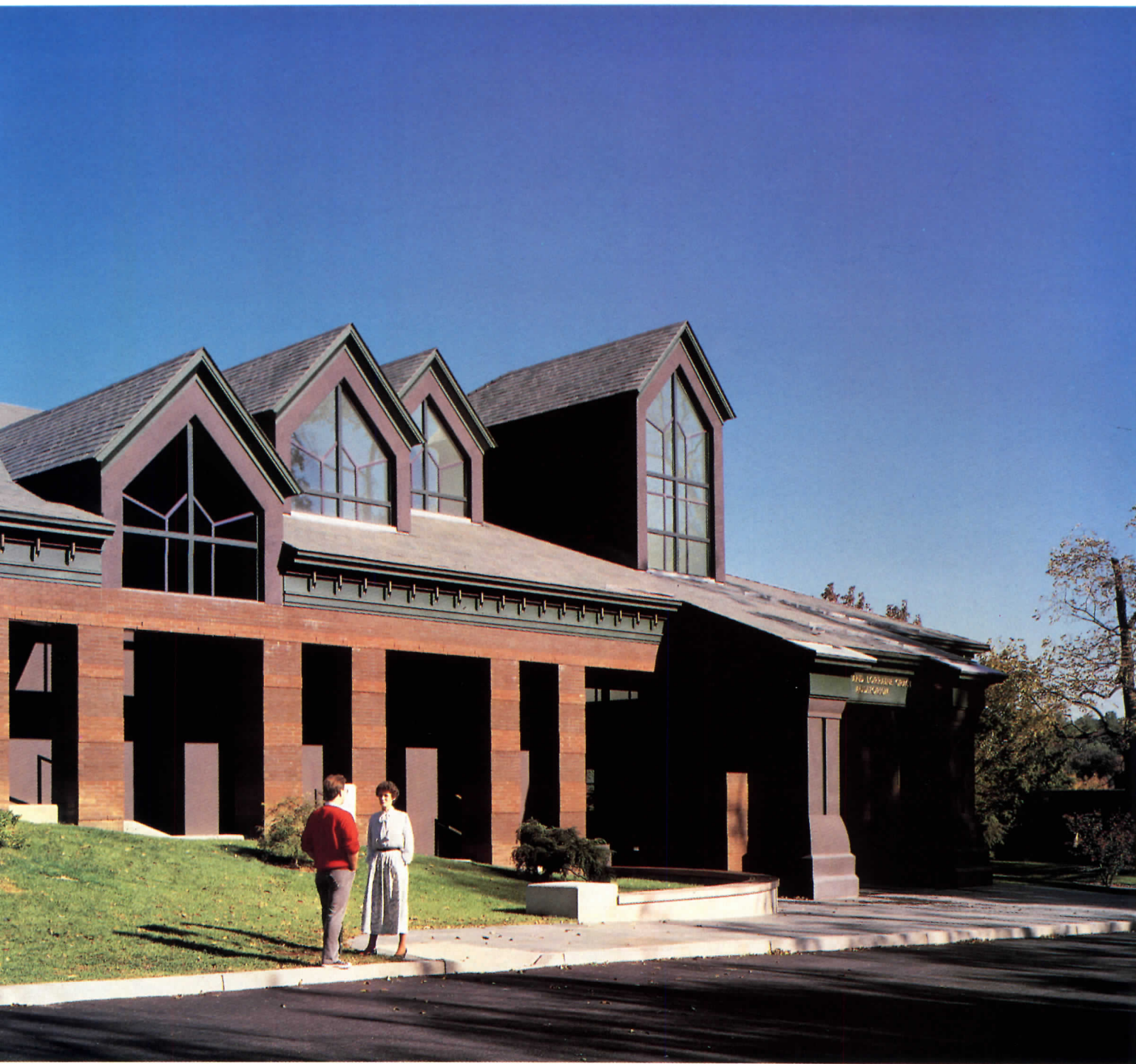
Above, a loggia running the length of the south facade provides shading in summer while the oversized dormers admit natural light to the lobby. Photo at far left shows east end and north elevation with a single dormer above the back entrance.
