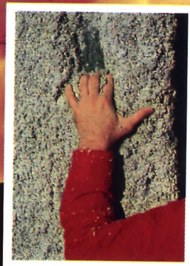
Mineral Wool Sprayed Fiber
