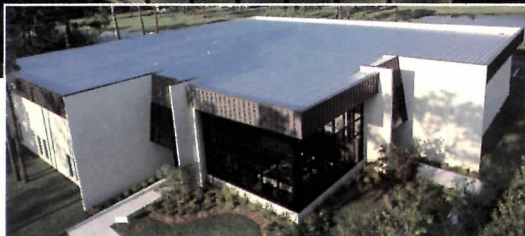
Owner: Countryside Cathedral, Clearwater, Fla. Design/Build Contractor: UNICO, Clearwater, Fla. Building System Manufacturer: Ceco Building Division, Southern Region, Columbus, Miss. Steel Material: Bethlehem Galvalume sheet
