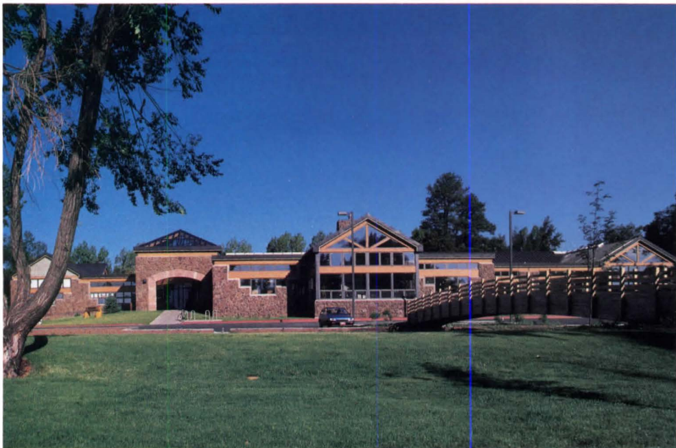
Left, a full view of the east side, with sandstone arch marking the entrance; the wooden footbridge crosses a stream. Interior views show concrete columns, three of the four fireplaces, and wooden beams and fan trusses. In photo at right, along east-west axis, linear skylight is detailed to ride over truss tips, and the rounded circulation desk is at far right.
