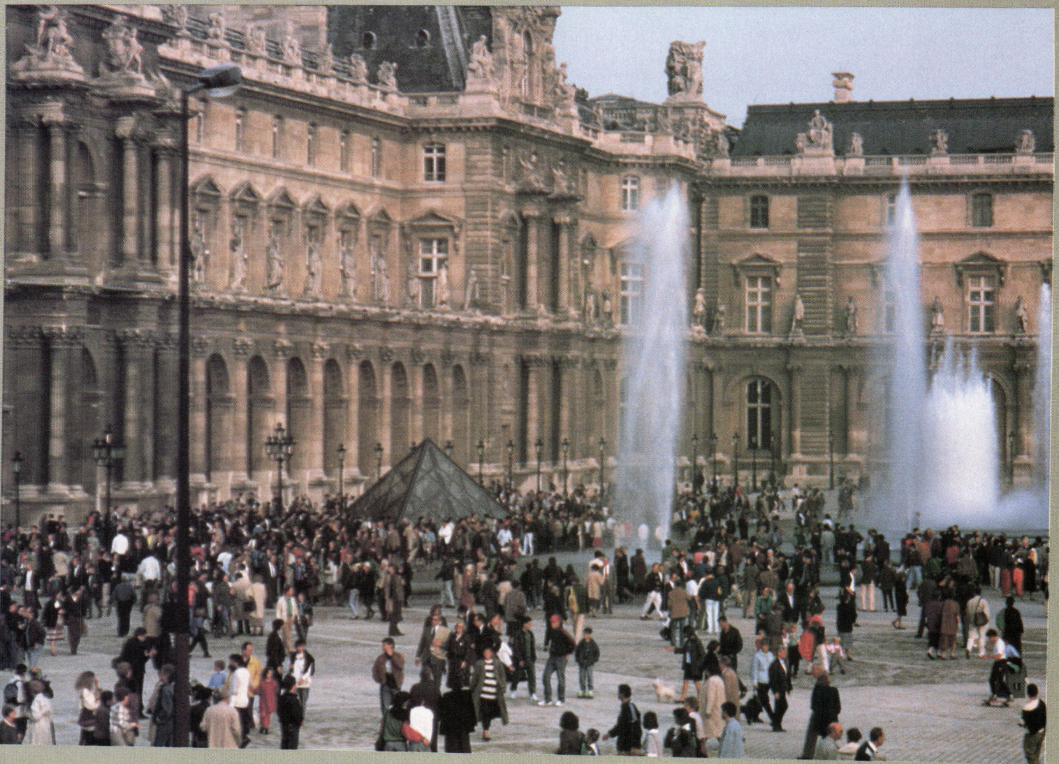
Above, a telescopic view into the northeast corner of Cour Napoleon showing one of Pei's small pyramids and the high fountains against the Louvre's Napoleon III facades. Each of the three small pyramids is 16 feet tall.
