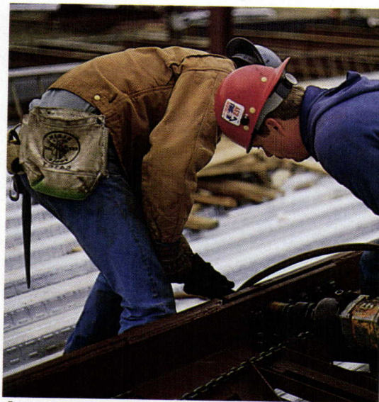
Joist sections are easily assembled on site.
