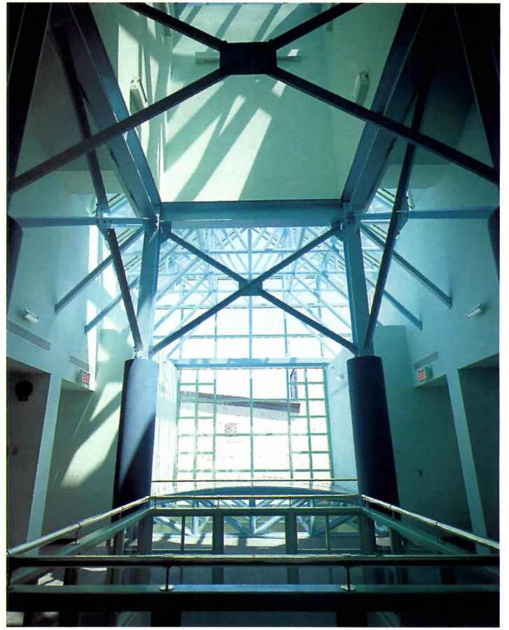
Three types of exterior skylights illuminate the building, as revealed in section (bottom left): a steel-braced glass pyramid, which tops a railing-encircled interior fiberglass skylight (below); a curved truss, fiberglass entryway skylight (bottom); and the insulated-glass panel and steel frame construction of the pitched roof (left).
