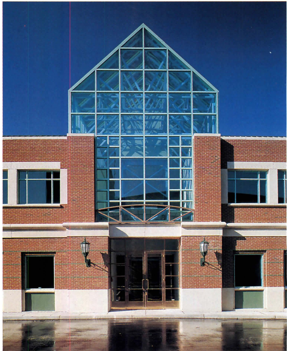
Pyramidal corner skylights punctuate the labor union's massing (left). A pitched-roof, insulated-glass skylight marks the entrance and exposes the building's steel frame (below).
