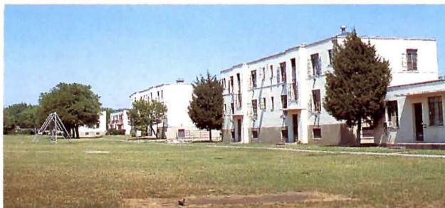
Recent view of the Cedar Springs public housing complex.
