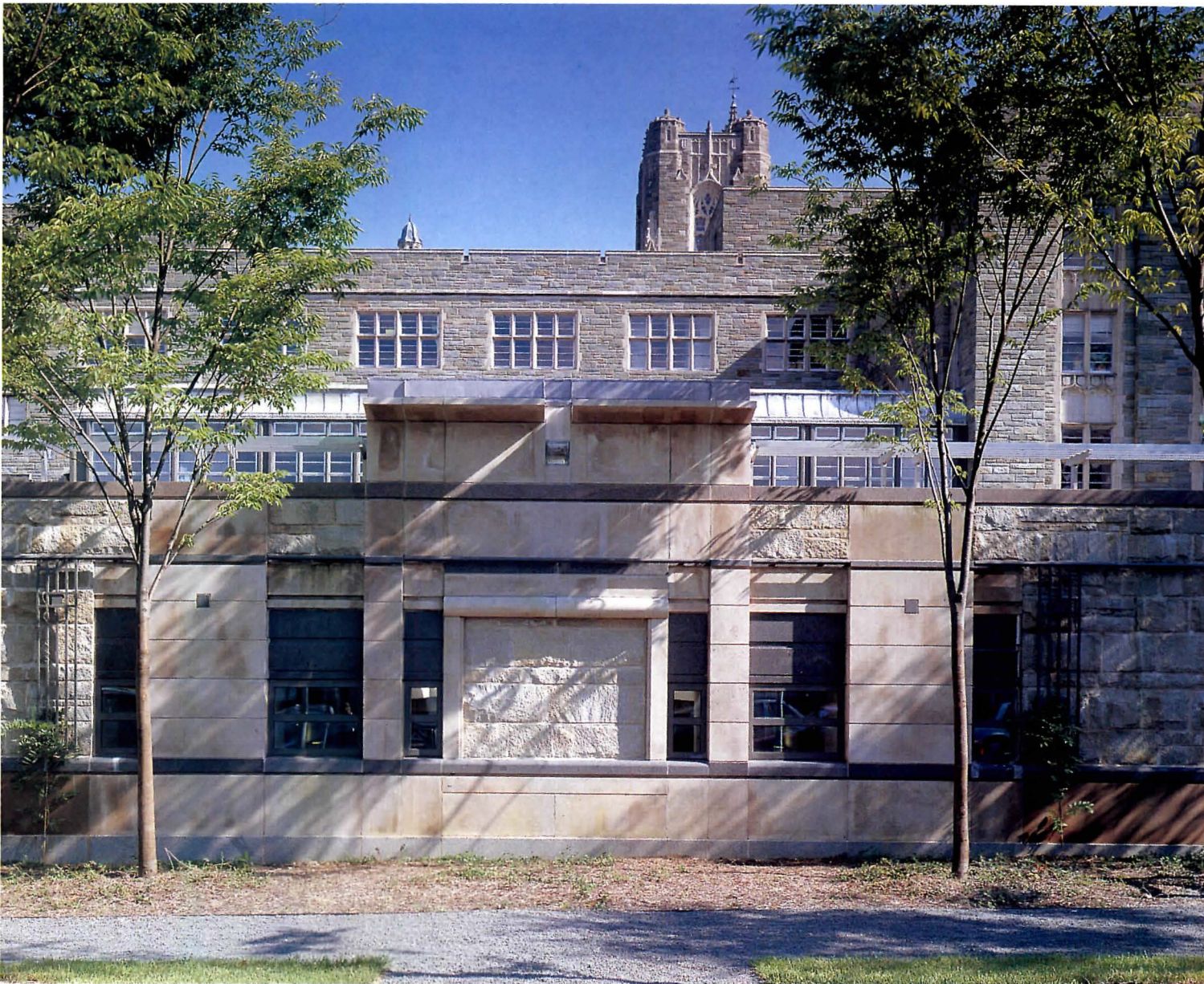
The architects treated the library's principal elevation on Nassau Street as a garden wall, articulating its surfaces with rhythmic compositions of limestone and granite in a variety of finishes (above), and wisteria-planted vertical trellises (facing page, top). They sliced the top of the turret (facing page, bottom) with a skylight to admit daylight.
