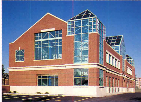
Pyramidal corner skylights punctuate the labor union's massing (left). A pitched-roof, insulated-glass skylight marks the entrance and exposes the building's steel frame (below).
