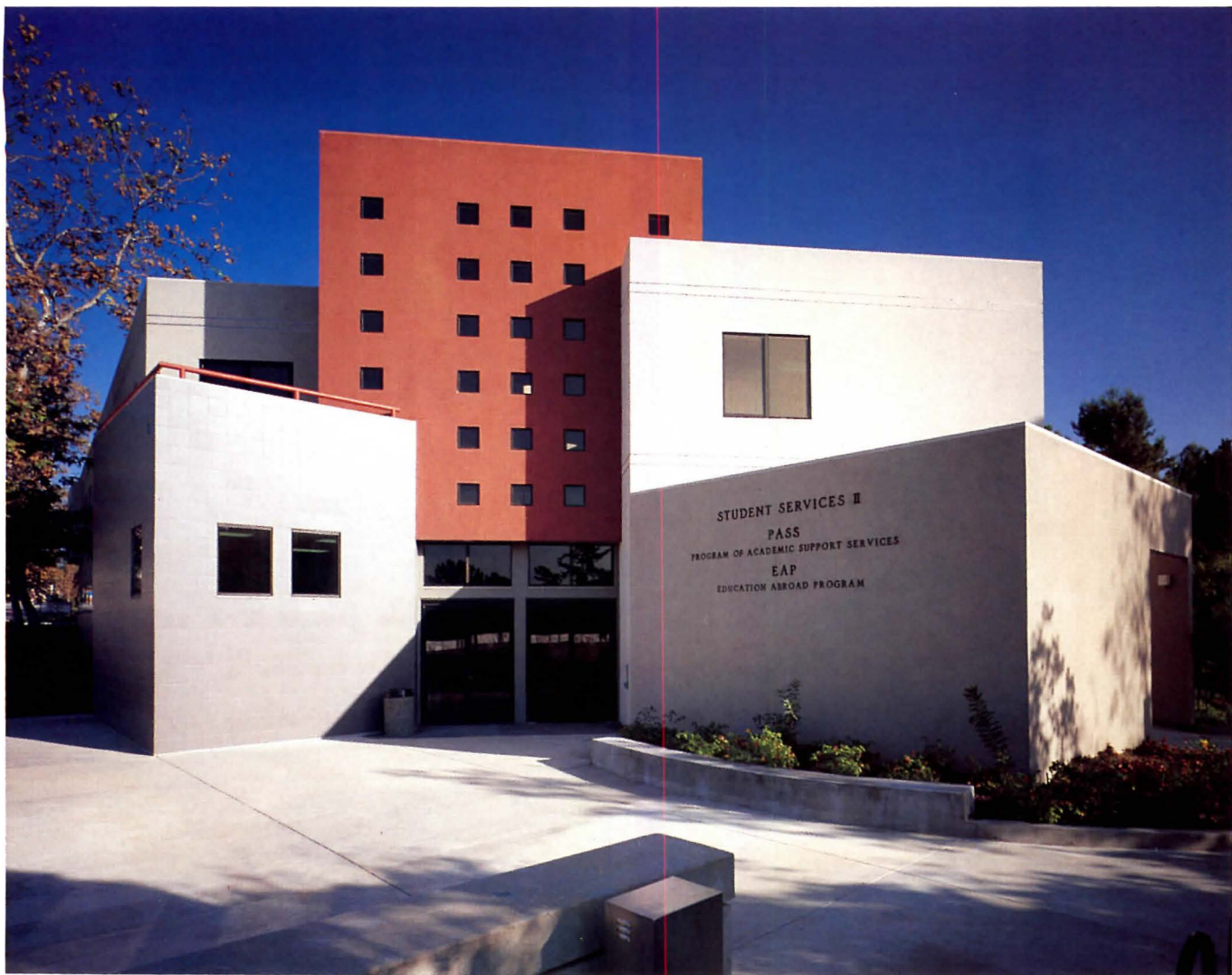
Student Services Addition Siegel Diamond Architects
