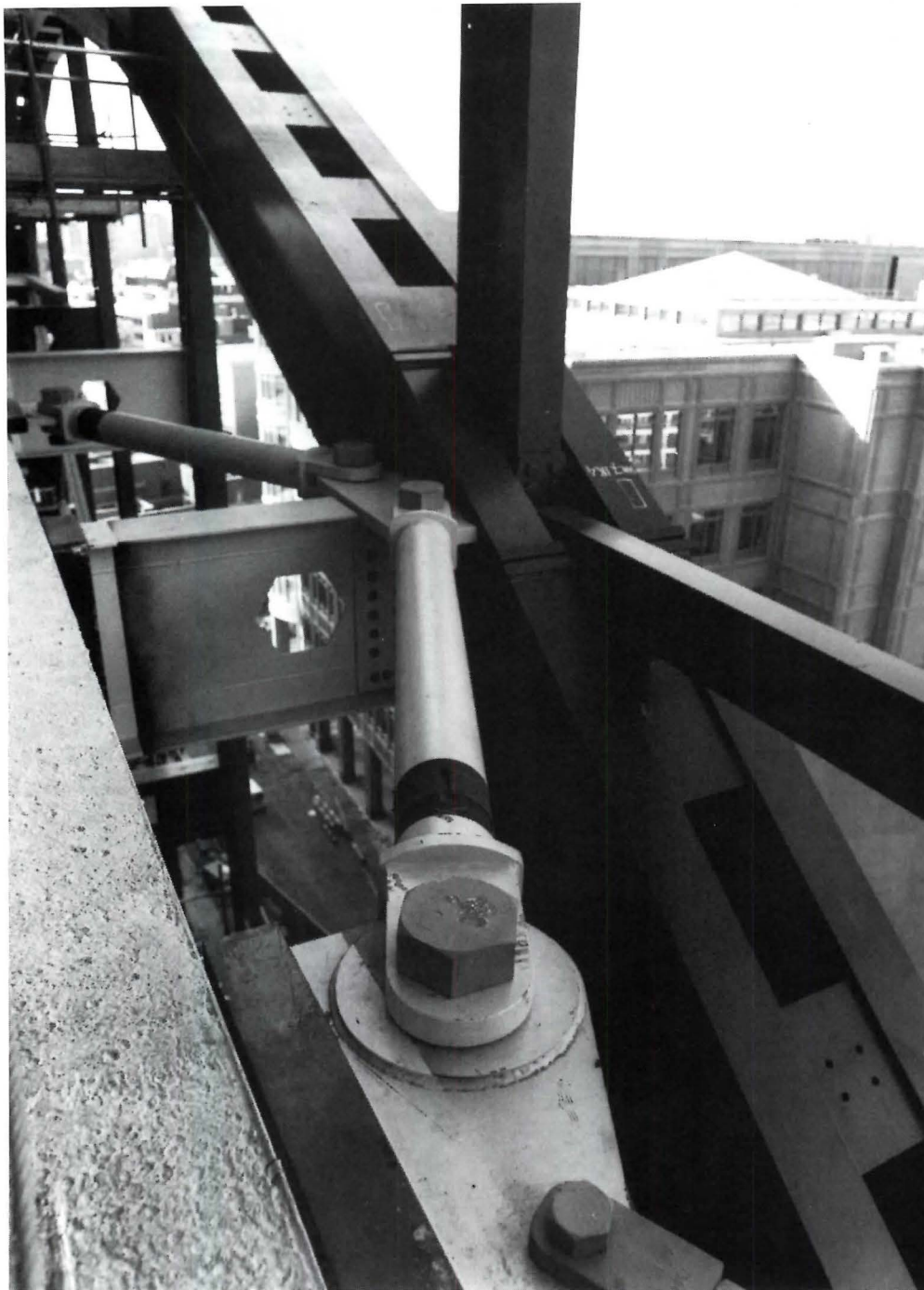
Struts (left) provide lateral support to the exterior frame by tying it back to interior girders. At the base of each arch the major structural elements join at a node (bottom left and below). Loads are then transferred to buttressed piers (above).
