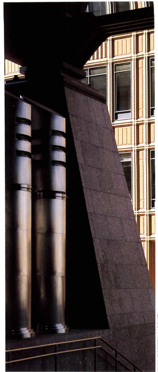
Struts (left) provide lateral support to the exterior frame by tying it back to interior girders. At the base of each arch the major structural elements join at a node (bottom left and below). Loads are then transferred to buttressed piers (above).
