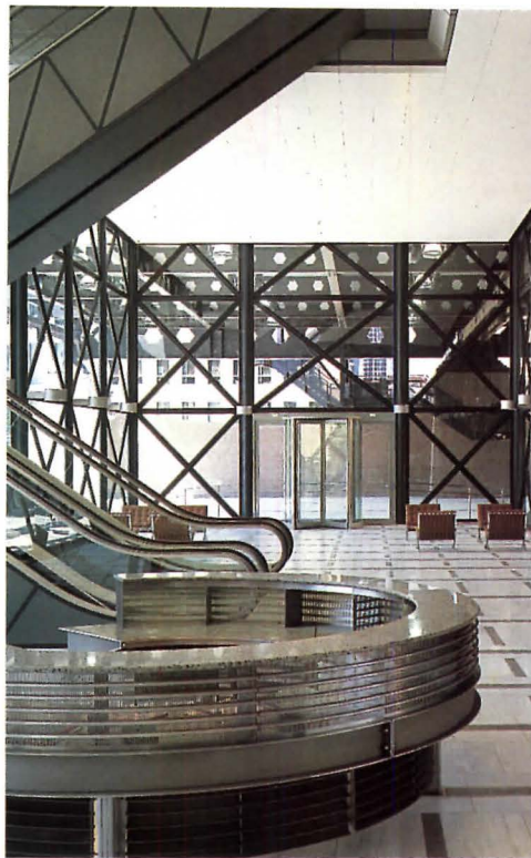
The lobby and elevators are enclosed in glass to create a sense of transparency (above), in contrast to the solid structural members. Interior arches are partially revealed in two
