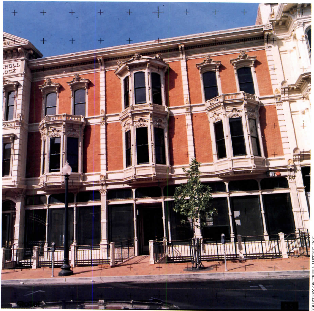
Accurate measurements equal to those obtained from calibrated cameras can be made from standard film exposures (above). Using the Rollei system, a grid of points is superimposed on the image, which can be taken from any angle, and a computer program will compensate for film and perspective distortions by digitizing the points.
