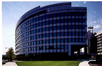
Bonneville Power Headquarters Portland, Oregon Zimmer Gunsul Frasca Partnership
