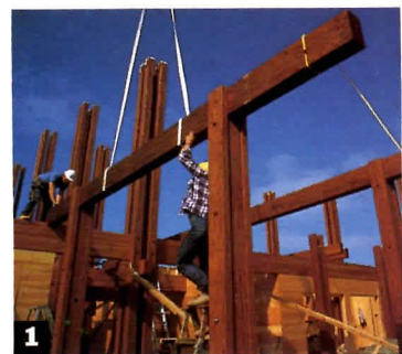
1. Vancouver architect Henry Hawthorne specified Parallam beams and columns manufactured of wood fiber and long strands of clipped veneer from MacMillian Bloedel Limited for a three-story, 20,000-square-foot research facility in British Columbia. Circle 413 on information card.
