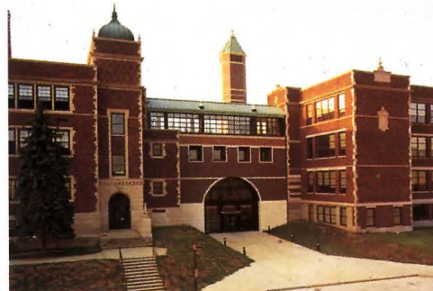
Renovation of Holmes High School Covington, Kentucky Burgess & Niple Limited, Architects
