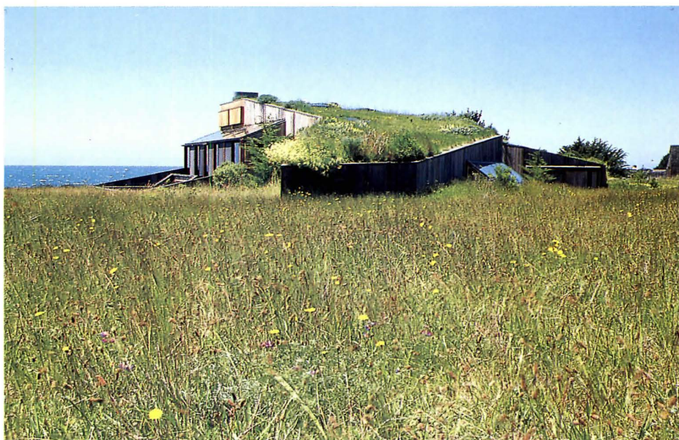
Incorporating indigenous plants and a sod roof (above), the earth-covered Brunsell house blends with the landscape (below).
