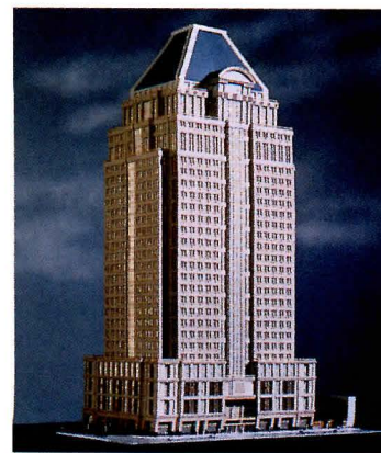
COMMERCE PLACE BALTIMORE, MARYLAND
