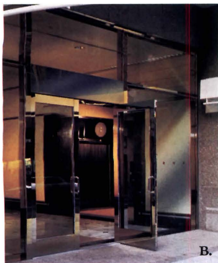
A. Freedom Square Building Cleveland, Ohio Architect: Ross C. Farro Glazing Contractor: Lorain Glass Co., Inc.
