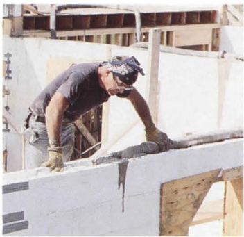
TOP: Insulated wall cavity modulates concrete's dehydration and thermal changes, diminishing risk of ruptures. ABOVE: Formwalls require minimal skill to assemble. Damaged portions can be repaired before concrete pour. RIGHT: Section through a typical wall constructed of stay-in-place formwork reveals steel ties and attachments.
