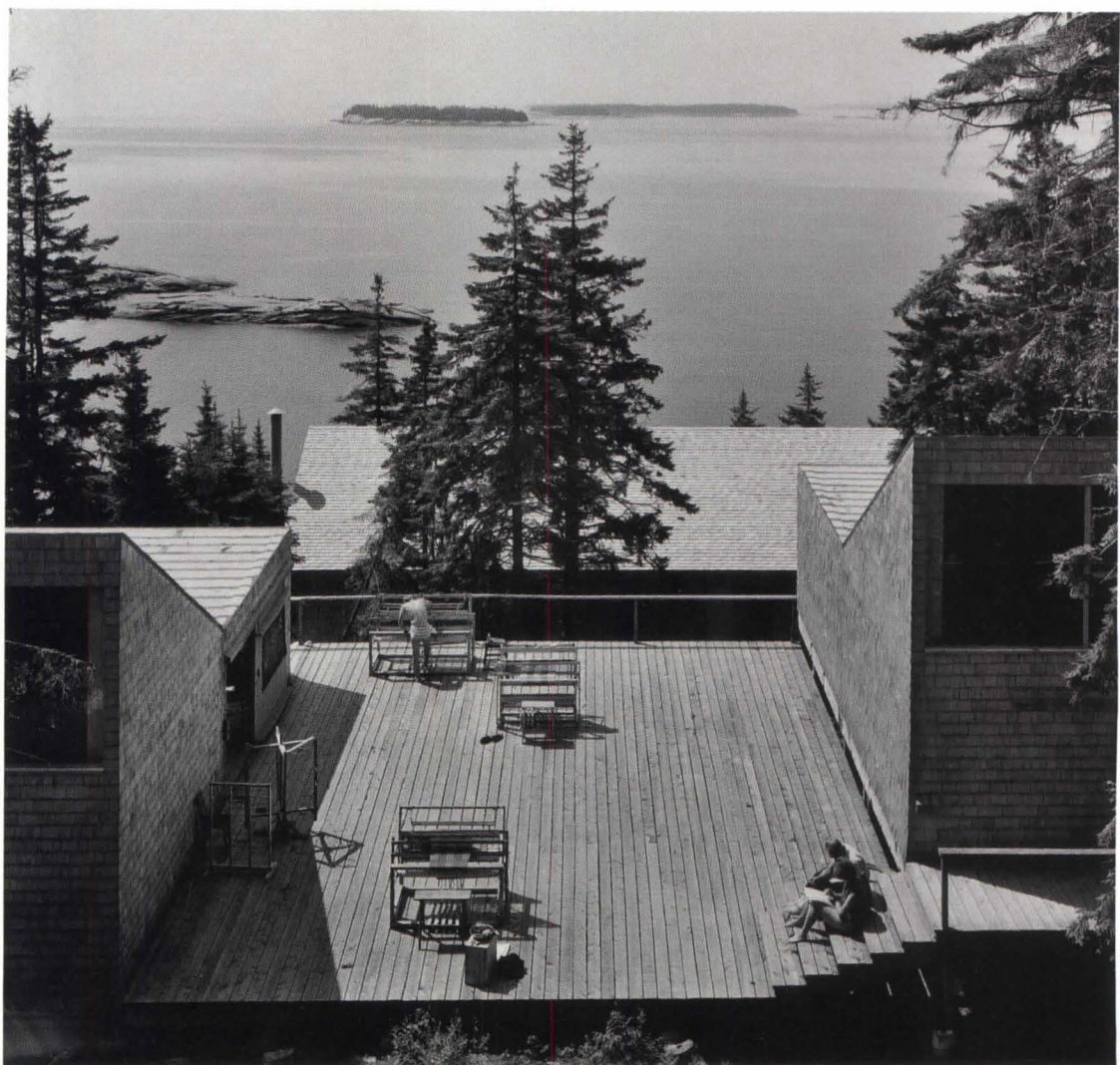
HAYSTACK SCHOOL: Barnes' 1961 complex integrates wood structures into landscape, offering coastal vistas.
