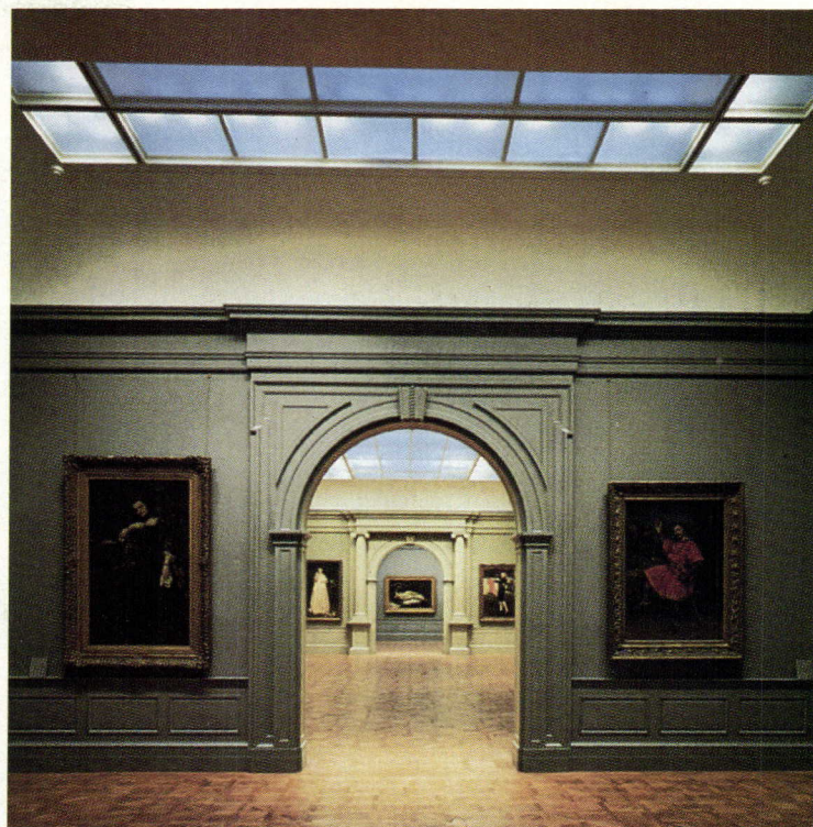
NEW GALLERIES: Plastered sheetrock and painted wood moldings.
