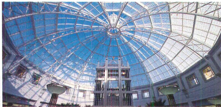
ROTUNDA: Fritted skylight reduces solar gain and increases thermal comfort.
