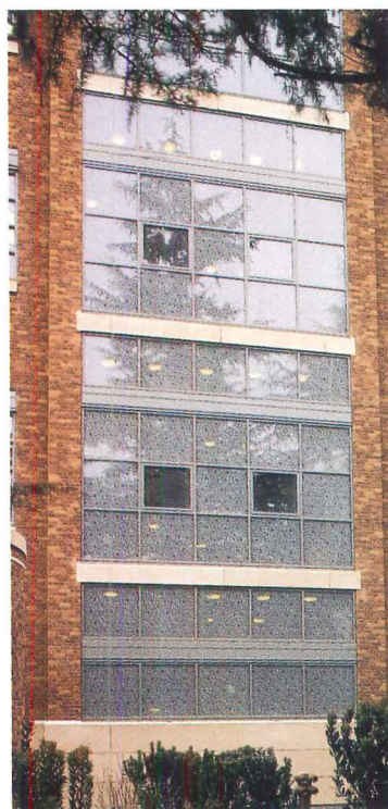
STAIR TOWER: Fritted windows.
