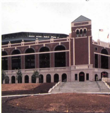
MASONRY SHELL: Concourse, offices.
