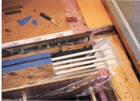
BEAM REPAIRS: Epoxy inserted over rods.
