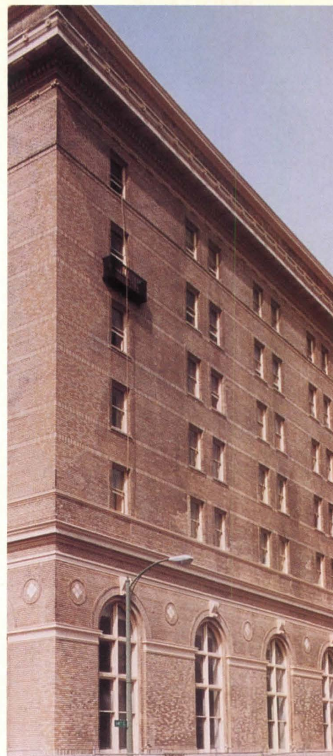
AFTER: Cracks in brick facade restored with epoxy.
