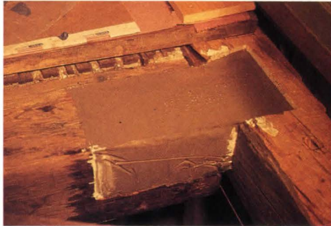
REPAIRED GIRT: Epoxy finished to resemble wood.
