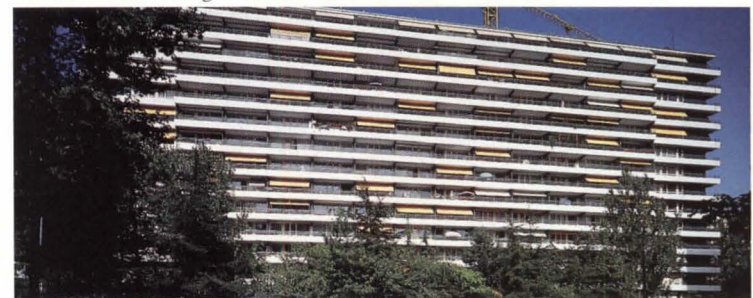
RUE NATIONALE: Apartment building renovation in Paris.
