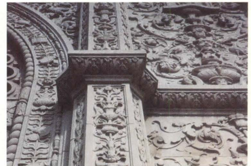
STONWORK: Reaffixed with steel pins and epoxy.
