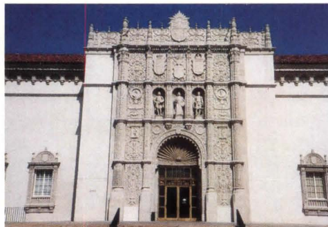
MUSEUM ENTRY: Stone entrance portal was repaired.
