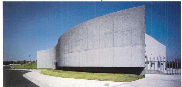
ALLEN & PARTNERS: Cast-in-place concrete forms curved wall of high school theater.
