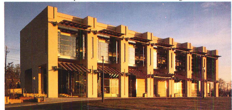
A.J. DIAMOND, DONALD SCHMITT: Precast concrete panels shade library interiors.
