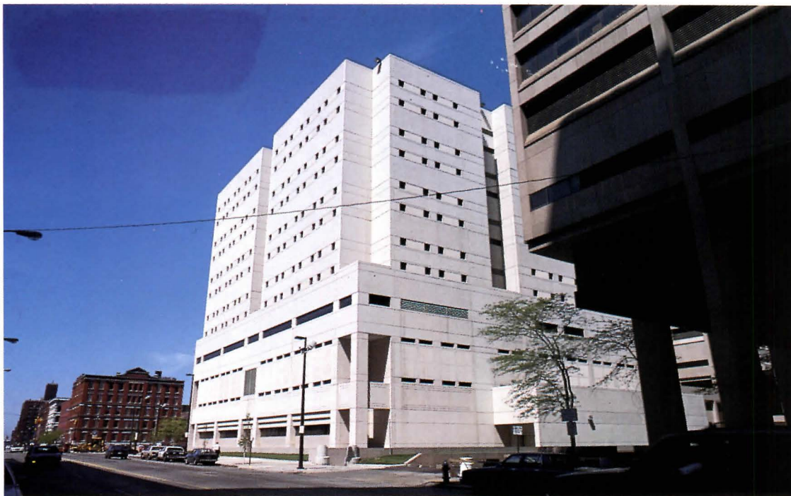
JAIL II: Clad in precast concrete, Cleveland's new high-rise jail is an alien presence in the heart of downtown.
