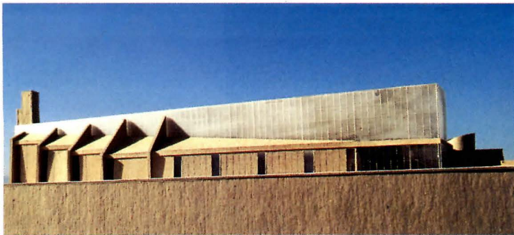
Central Plant With Cogeneration University of California Davis Medical Center Sacramento, California Siegel Diamond Architects
