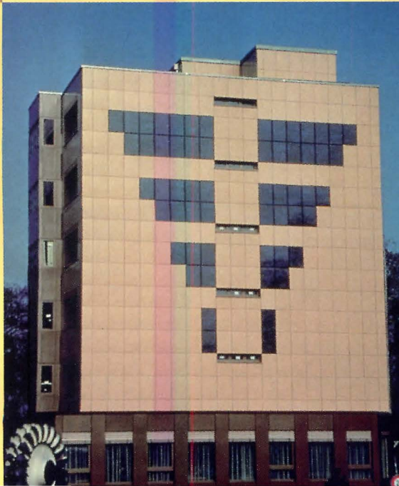
Utility Company Headquarters: Photovoltaic façade
