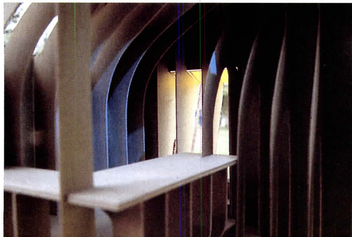
Detail of interior fins
