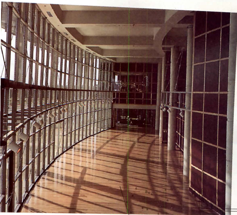
Curtain wall structure comprises clear, anodized aluminum framing members and insulating reflective glass panels that consist of two 1/4-inch-thick sheets separated by 1/2-inch air space.
