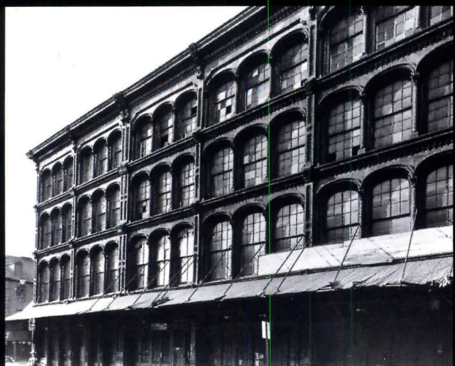
Five-bay, cast-iron facade of 1869 G. Fava Fruit Company Building (below) was reassembled into stepped configuration (above).
