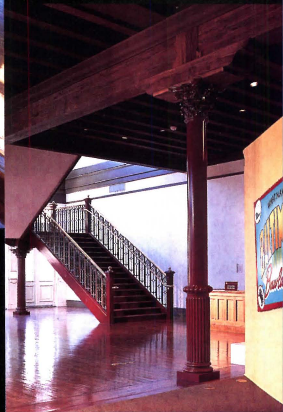
Interior steel columns are encased by cast-aluminum wainscoting and Corinthian capitals. They are topped by heavy timber beams and joists to recall detailing of a Venetian palazzo and exposed wood structure of original warehouse. Beams measuring 13 inches wide by 24 inches deep conceal lighting, electrical wiring, sprinklers, and ductwork between members.
