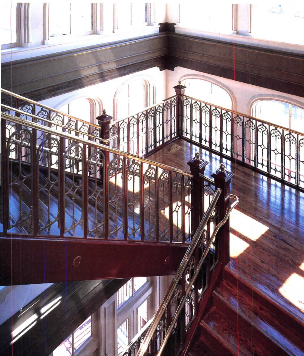
Grand staircase incorporates cast-aluminum balustrade fabricated by Baltimore ironworker Paul Peranio.
