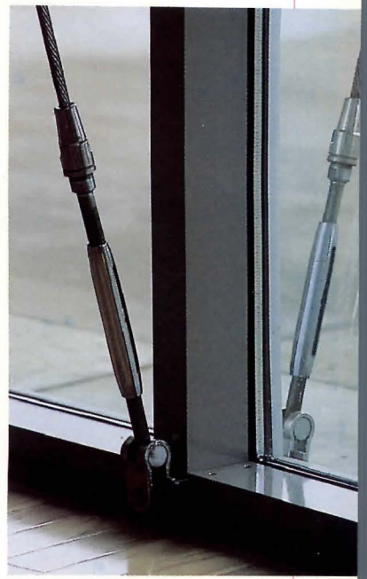
Supplemental steel cables and frames maintain 5 3/4-inch-deep aluminum framing members.
