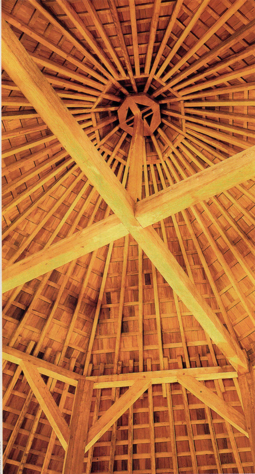
In keeping with the original, most of the barn is built of southern yellow pine, including the large king-post truss.
