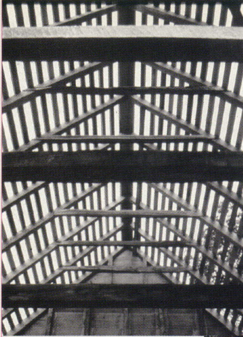
Oak rafters and beams of twin corn cribs are hand-sawn.
