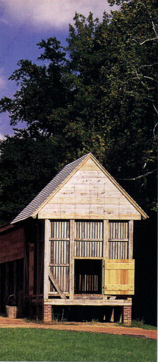
Quinn Evans's recreated treading barn at Mount Vernon (center) is flanked by corn cribs to store feed and stables that once housed horses, oxen, and mules.
