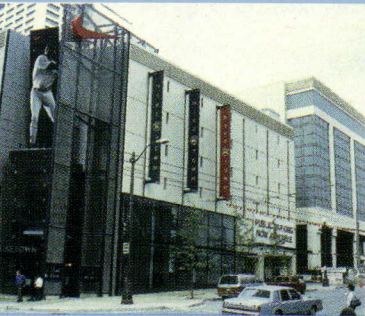
Seattle's Niketown store is topped by parking garage.
