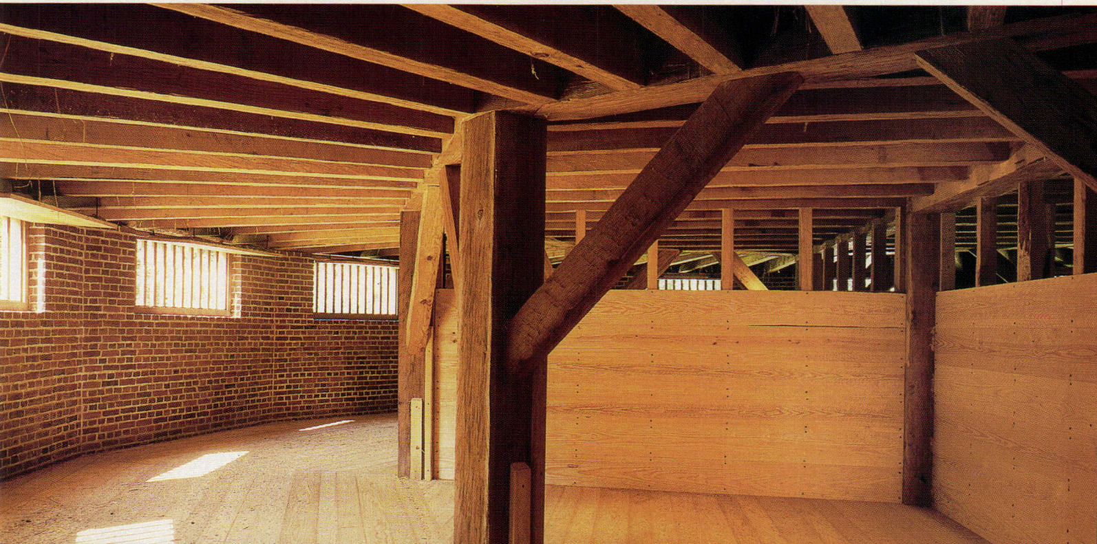
Sturdy white oak was harvested from the present-day Mount Vernon estate and applied to form the treading floor of the upper level (facing page, left). Oak was also used in critical structural members such as lower-level columns (below). Rafter details (facing page) show decorative ends common to period outbuildings for the gentry and overlapping rafters notched into the top plate of the inner octagon.
