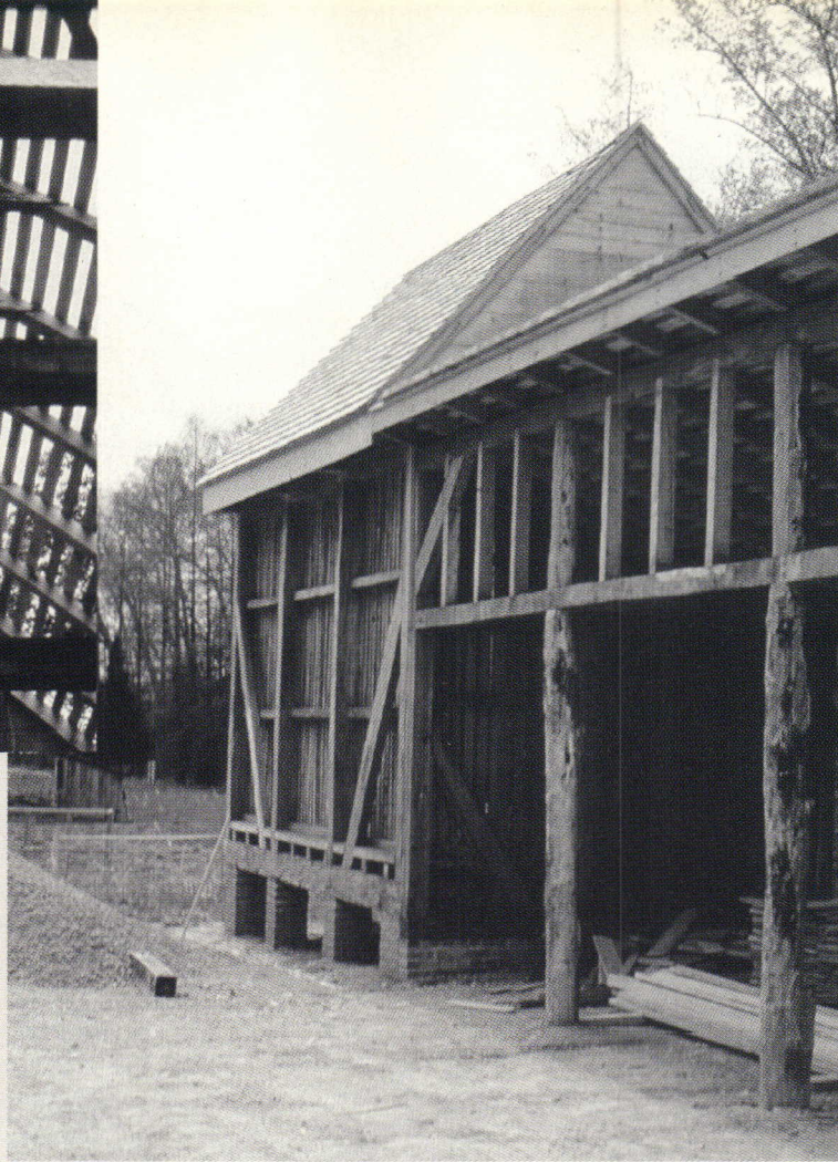
Original documentation of corn cribs and stables was limited to one plan by Washington, so their construction is more conjectural than the barn's. Using similar structures in the region as models, Quinn Evans interpreted two different periods—1780 and 1795—reflecting significant advances in construction.
