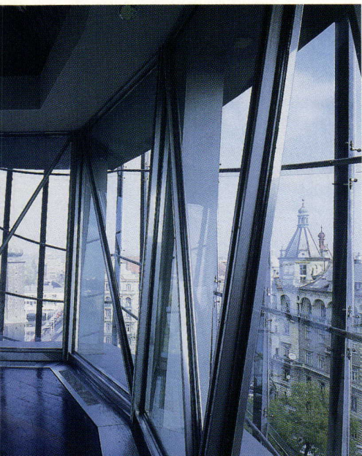
Ginger's top floor, with two glazed membranes, projects beyond the body of the main structure to afford sweeping city views.
