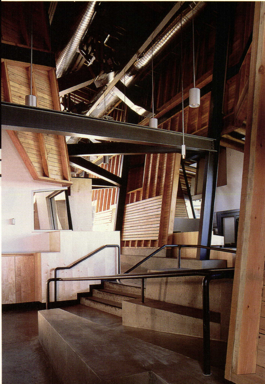
Entrance to classroom is marked by steel structure and maple plywood student lockers (above). Basic building systems are visible at juncture of library, technical center, and computer room (right).
