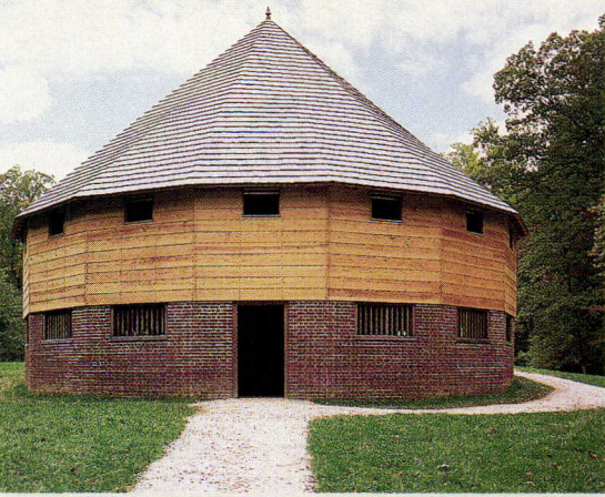
Lower-level walls are built of hand-molded brick for structural stability and security. Rear view (left) shows entrance to lower-level granary. To ensure dry conditions in the lower level, a mud slab was poured beneath the building and a modern drainage system installed (section below).
