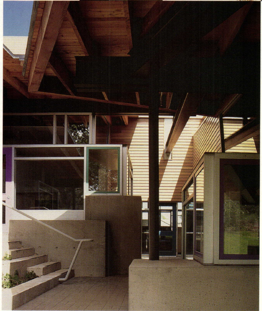
Porch (left) doubles as outdoor play area in British Columbia's rainy climate. Classroom pods are surrounded by vegetation with views of rocks and oak trees (top). View between classroom pods reveals dynamic material assemblies (above).
