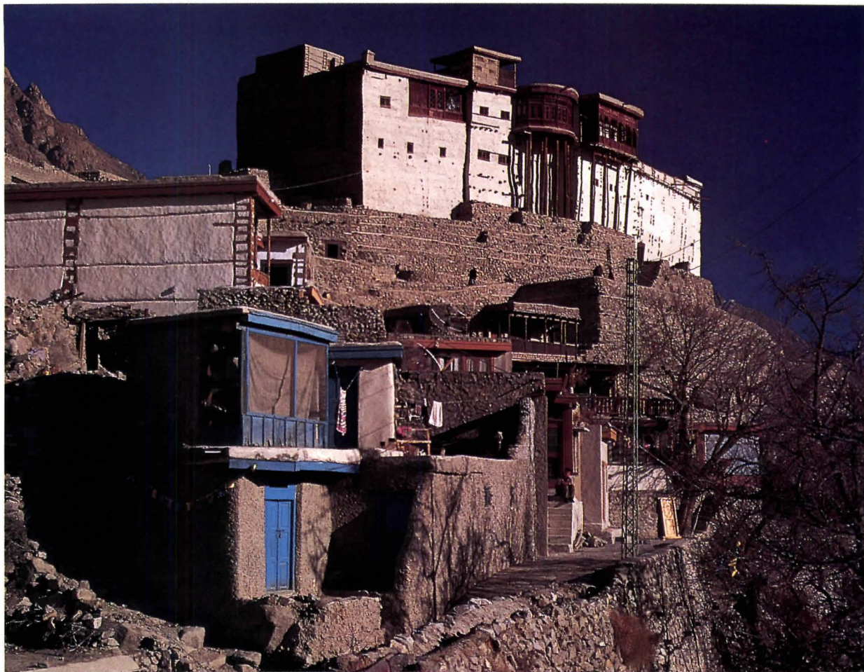
Central defensive tower evolved over centuries into mir's feudal palace and bastion, built of mud and stone. Victorian-style balcony and bay window, added this century, echo British colonial buildings. Historic structures cling to fort's steep slope; traditional stone irrigation channel is visible in foreground.
