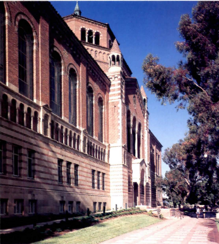
Concrete shear walls reinforce perimeter.
