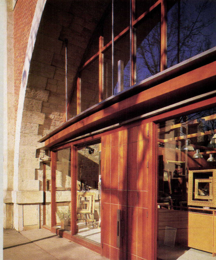
Bowed beam of storefront expresses optional mezzanine level. Transom window, set nearly two feet behind lower storefront panels, casts deep shadows that accentuate vaults' mass without decreasing rentable floor space.
