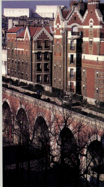
Railroad viaduct supports verdant garden.
