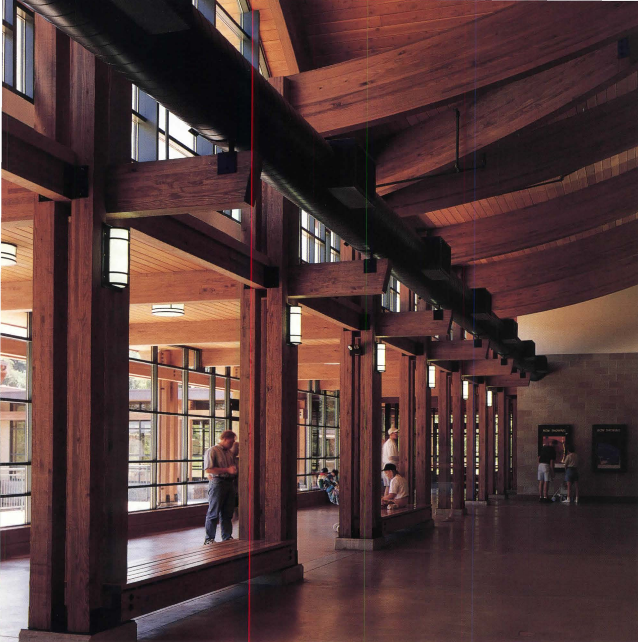
Adjoining artificial pond in sprawling Swope Park, pavilion's curved copper roof and cedar shingles create quiet yet visible entry to zoo (previous pages). Curved glulam beams and southern pine post-and-beam structure (left) create rustic feel in lobby of IMAX theater.
