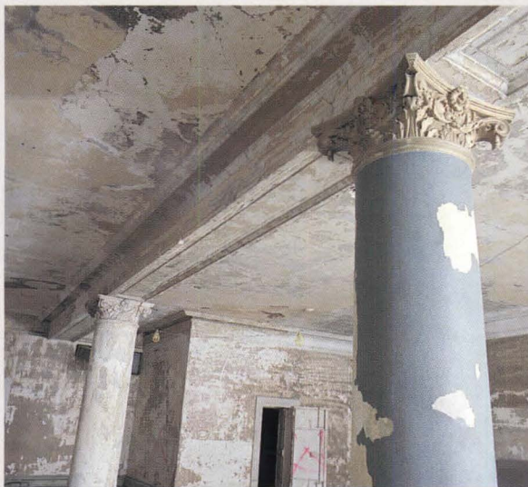
Crumbling plaster of columns and walls (above) was restored; space was converted into multi-purpose room (above right). Energy-efficient lighting is mounted above ceiling soffits.
