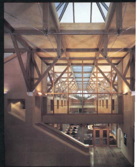
Wooden trusses braced by steel tension cables crown entry lobby.
