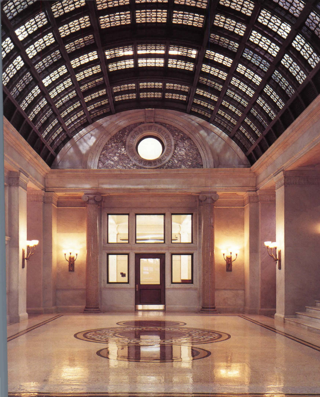
Refurbished skylight admits diffused daylight into central lobby. Existing gutters along edge of vault conceal new air ducts.
