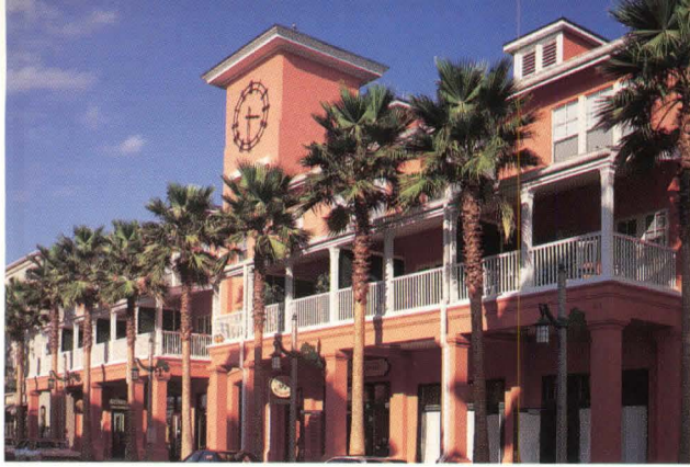
Apartments top stores along downtown streets.
