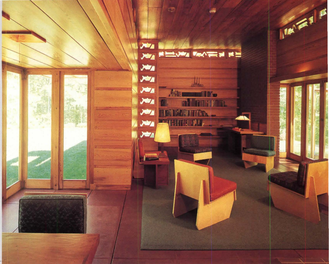
Before Quinn Evans' reconstruction, interior masonry and floor in living room (above) were visibly worn. Architect replaced masonry, refinished cypress ceiling panels, and poured new color-matched concrete floor. Furniture is mostly original to 1941 house.
