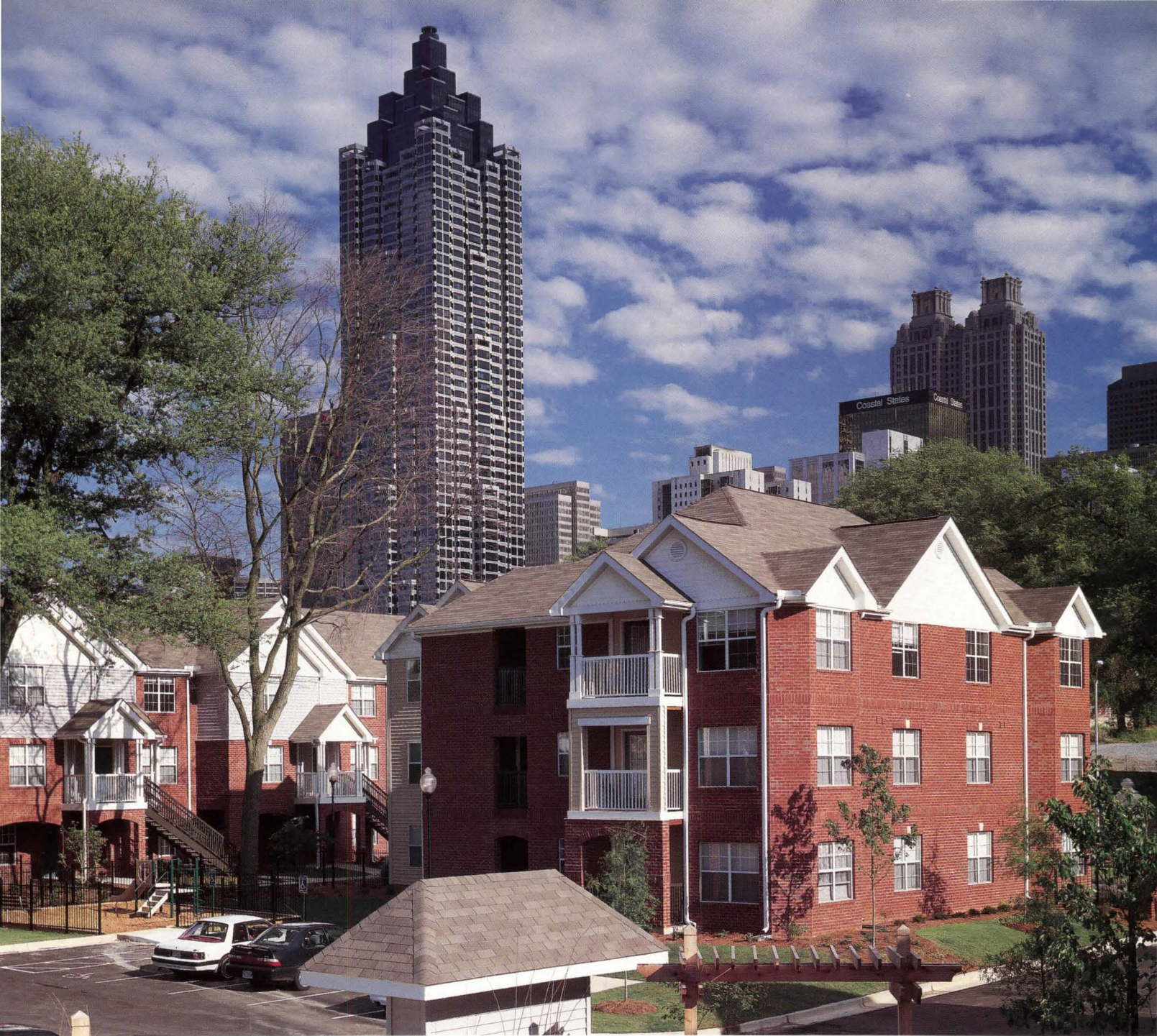
First completed units of Centennial Place direct sight lines from individual entrances toward the street, emulating Atlanta's traditional neighborhoods of wood-framed houses. Parking, however, is sequestered between buildings rather than on the street, following a suburban pattern.
