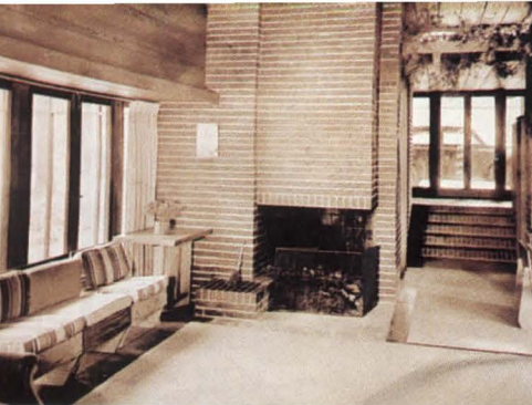
Before Quinn Evans' reconstruction, interior masonry and floor in living room (above) were visibly worn. Architect replaced masonry, refinished cypress ceiling panels, and poured new color-matched concrete floor. Furniture is mostly original to 1941 house.
