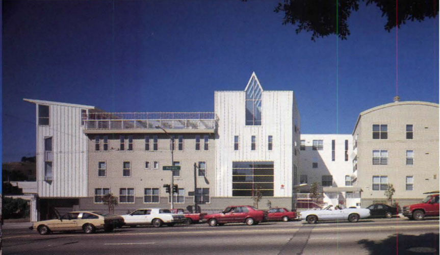
Four-story Good Samaritan Community Center is divided into community center (left) and a gray, bow-roofed structure containing apartments (right). More housing units are contained in bar building at rear of site. Flats occupy ground floor, and two-story apartments are located on top three floors, accessible from third-floor corridor (axonometric).
