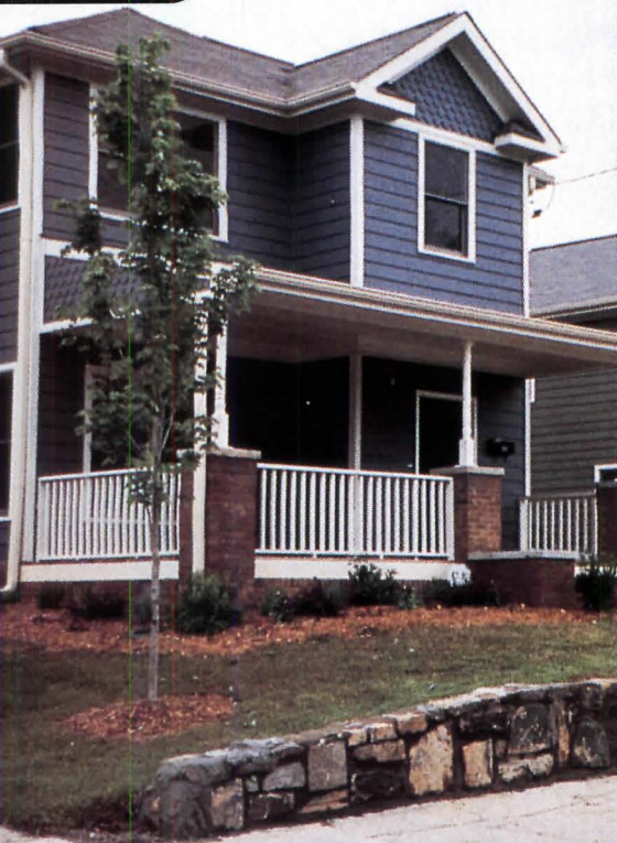
Construction in Atlanta's Martin Luther King, Jr. Historic District received a 1997 National Trust preservation award.
