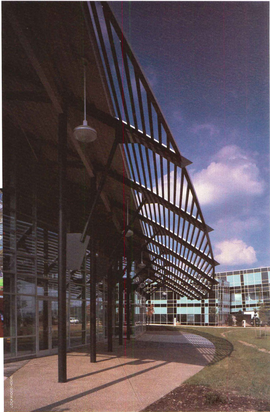
Cafeteria roof (facing page, left) curves over south end of Building 3. South entrance to Building 3 (facing page, right) combines material palettes of Buildings 1 and 2. Cafeteria interior (above left) features open web trusses, exposed HVAC, and abundant daylight. Open steel lattice sunshade on south facade of Building 3 (above right) screens cafeteria from direct sunlight.
