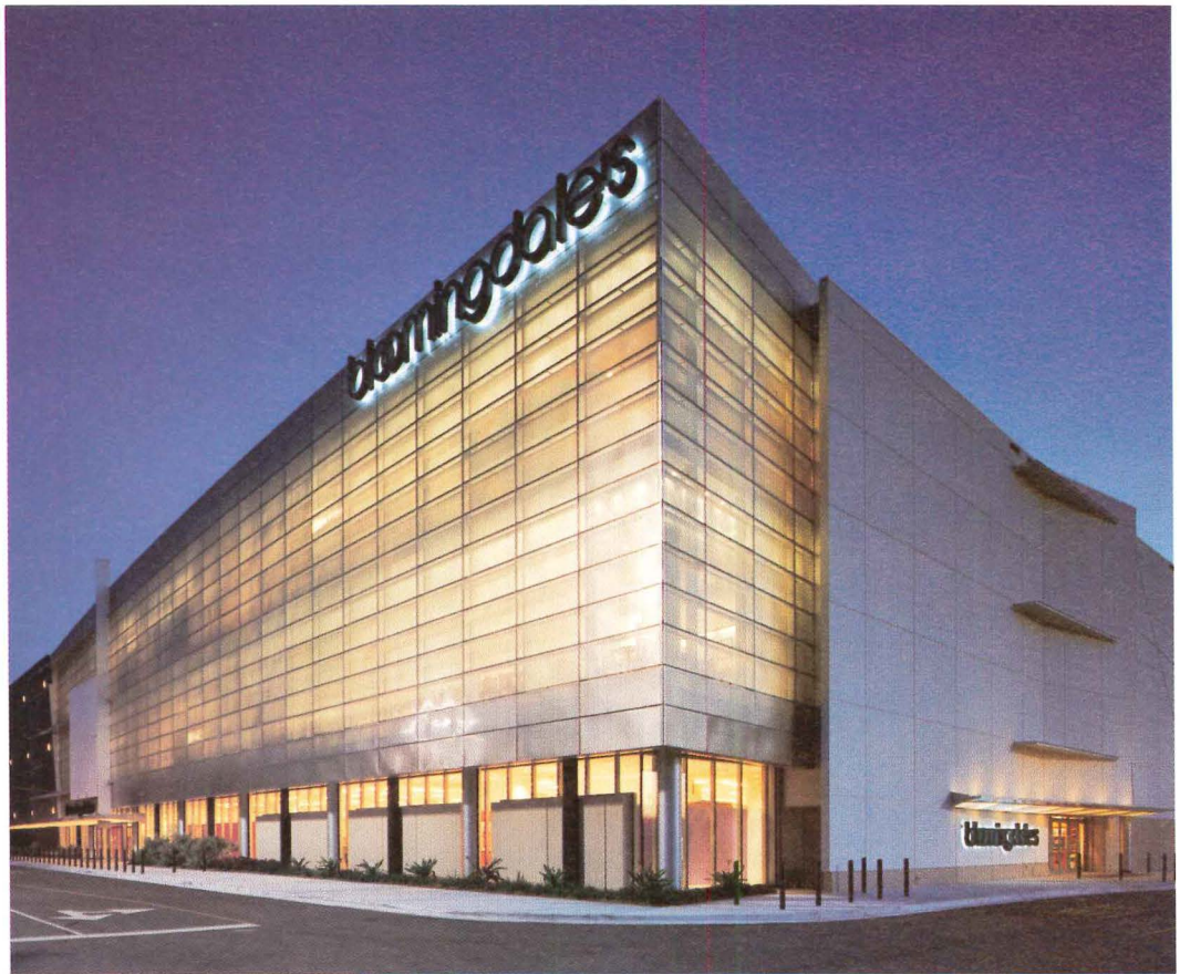
Aluminum fins and steel channels distinguish Bloomingdale's windowless south facade (facing page) from conventional department store. Perforated stainless steel panels project from curtain wall mullions (above). Modernist store (right) contrasts with adjacent Disneyesque food court building.
