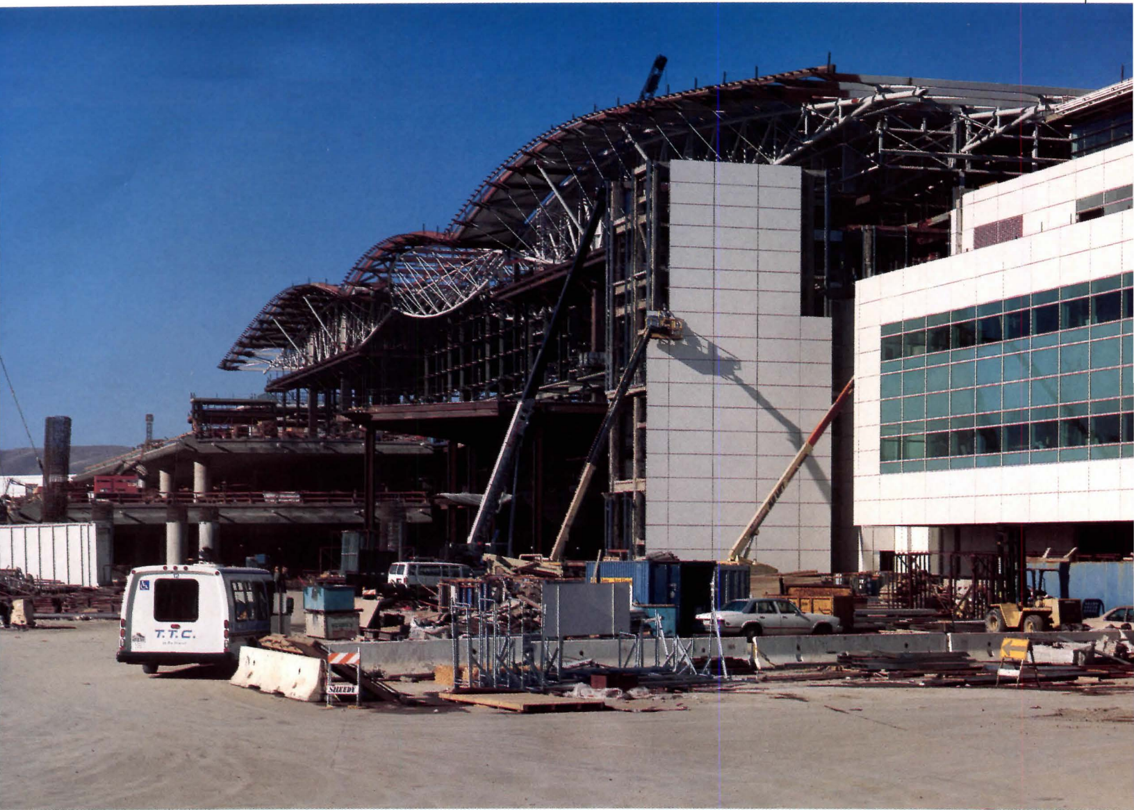
Truss system of new airport terminal, now under construction (above), spans 840 feet across main hall and roadway. Daylighting control includes skylights along main roof truss lines (below right); light reflected off sloped lower roof of concourse into terminal (below left); and, on west-facing window wall (facing page), clear glass, translucent patterned fritted glass, and metal brise-soleil.
