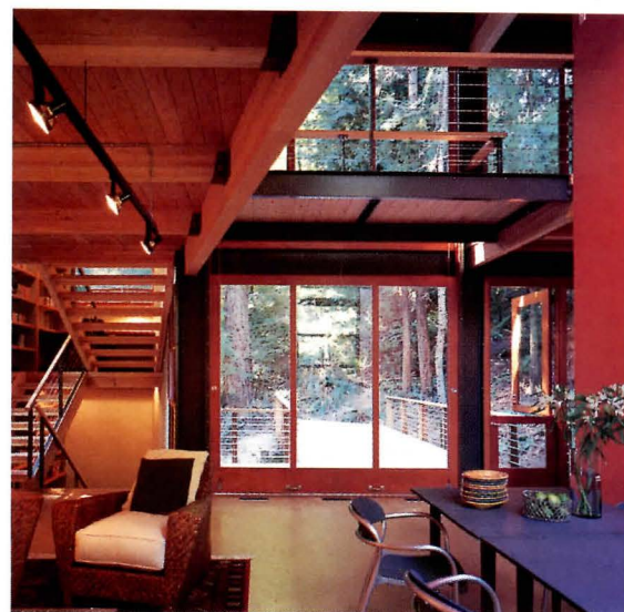
Rear facade (opposite page), with steel moment frame, provides full-height windows for third-floor living spaces and top-floor master bedroom suite. Inside, 3-panel glass door at deck (above) slides up vertically to height of balcony.
