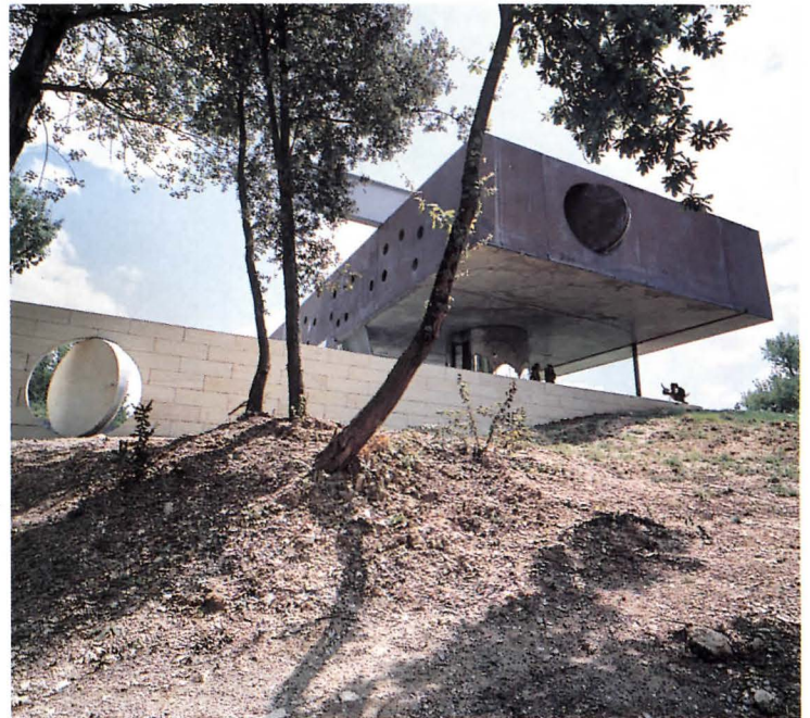
Concrete box (above) seems to float above concrete courtyard wall with stone veneer; box is supported underneath by stainless steel-clad concrete stair enclosure and from above by 36-inch-tall cantilevered steel beam.
