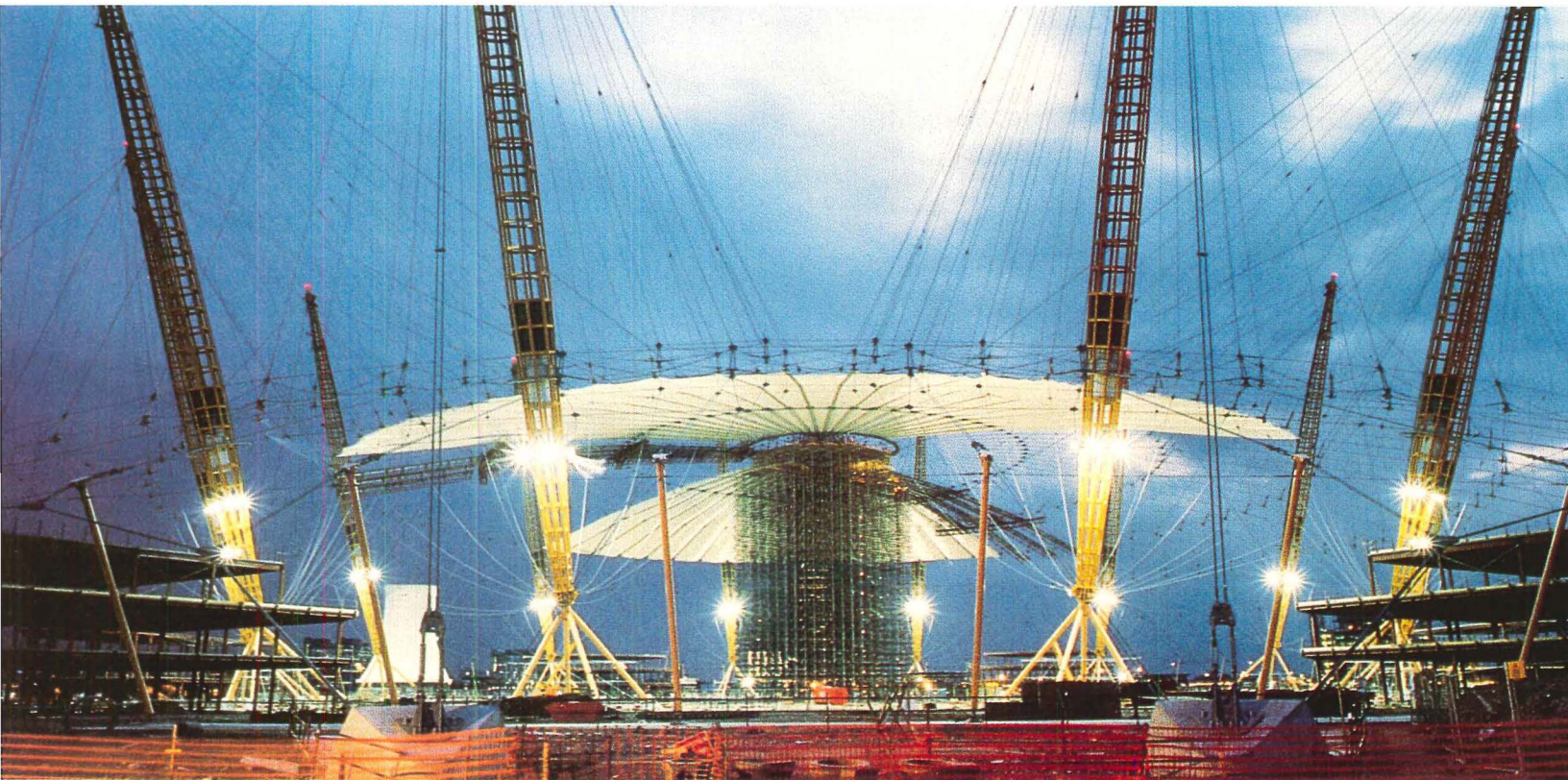
Wishbone nodes connect circumferential cables to pairs of radial cables that form a netting (above), which will hold tensioned membrane panels. Scaffolding (below) made of 44 miles of steel tubing gives workers access to cable network. Aerial view (opposite page) looks over dome on 181-acre site next to River Thames.
