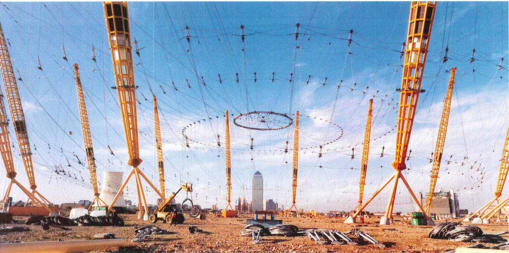
Wishbone nodes connect circumferential cables to pairs of radial cables that form a netting (above), which will hold tensioned membrane panels. Scaffolding (below) made of 44 miles of steel tubing gives workers access to cable network. Aerial view (opposite page) looks over dome on 181-acre site next to River Thames.
