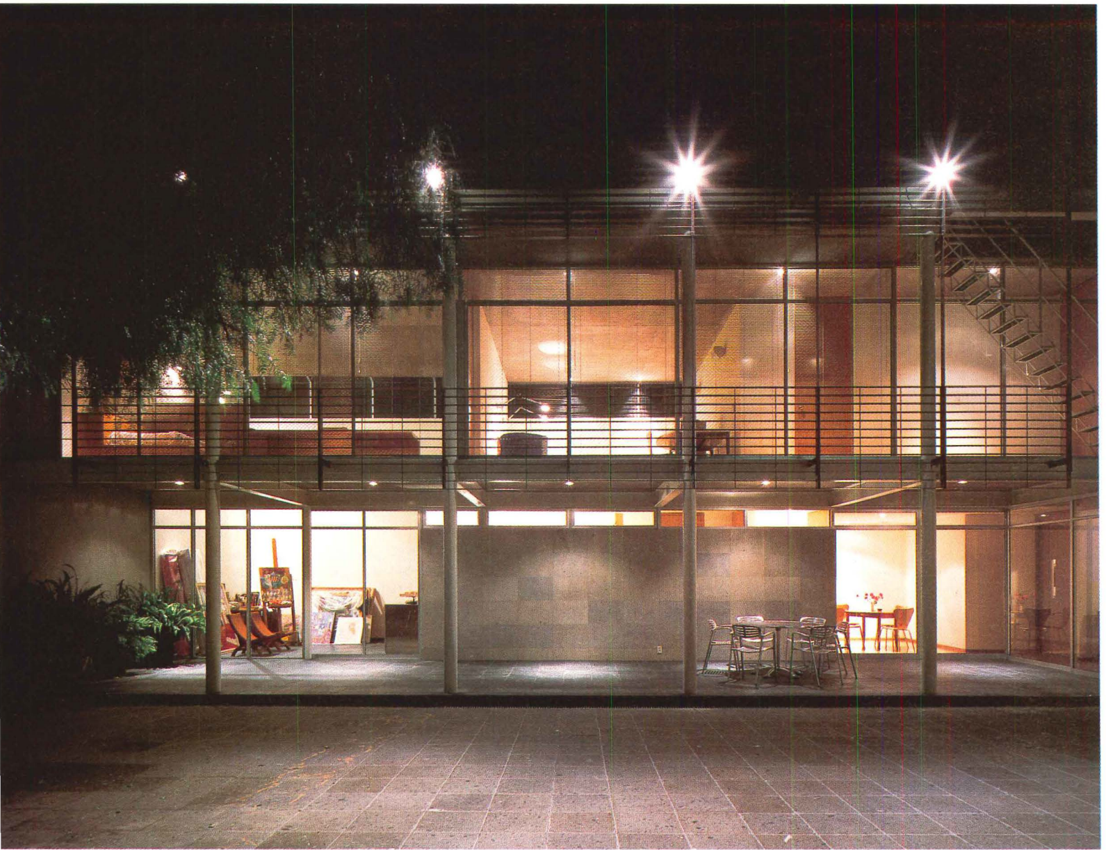
At night, facade of bedroom wing (above) all but disappears. Screened by steel grilles, glazed facades reveal narrow interior rooms, including double-height painting studio and loft (at left); master bedroom above service quarters (at center); and bedrooms atop breakfast area (at right). Clerestories along rear wall of loft and master suite edit views out to surrounding valleys.
