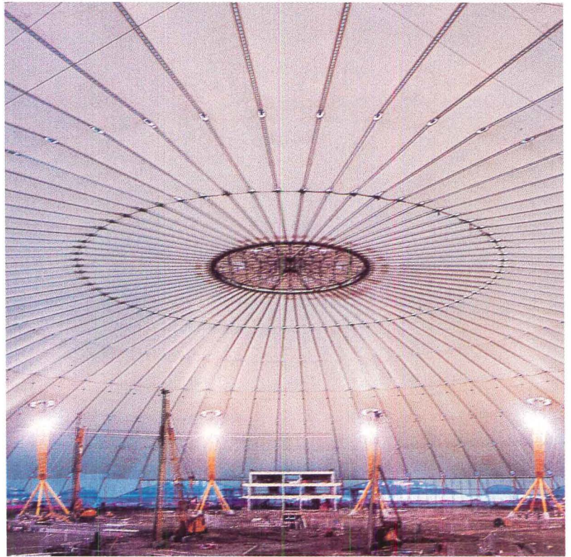
Perspective from dome's interior floor (above) provides expansive view of completed Teflon-coated fabric panel installation. Computer rendering (below) shows 12 exterior service structures that feed six internal physical plants. Abseilers (left) on top of dome cable network unfurl tensioned membrane panels, each weighing just under 1 ton.
