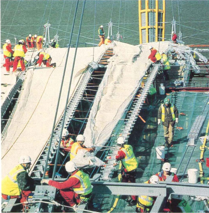
Perspective from dome's interior floor (above) provides expansive view of completed Teflon-coated fabric panel installation. Computer rendering (below) shows 12 exterior service structures that feed six internal physical plants. Abseilers (left) on top of dome cable network unfurl tensioned membrane panels, each weighing just under 1 ton.
