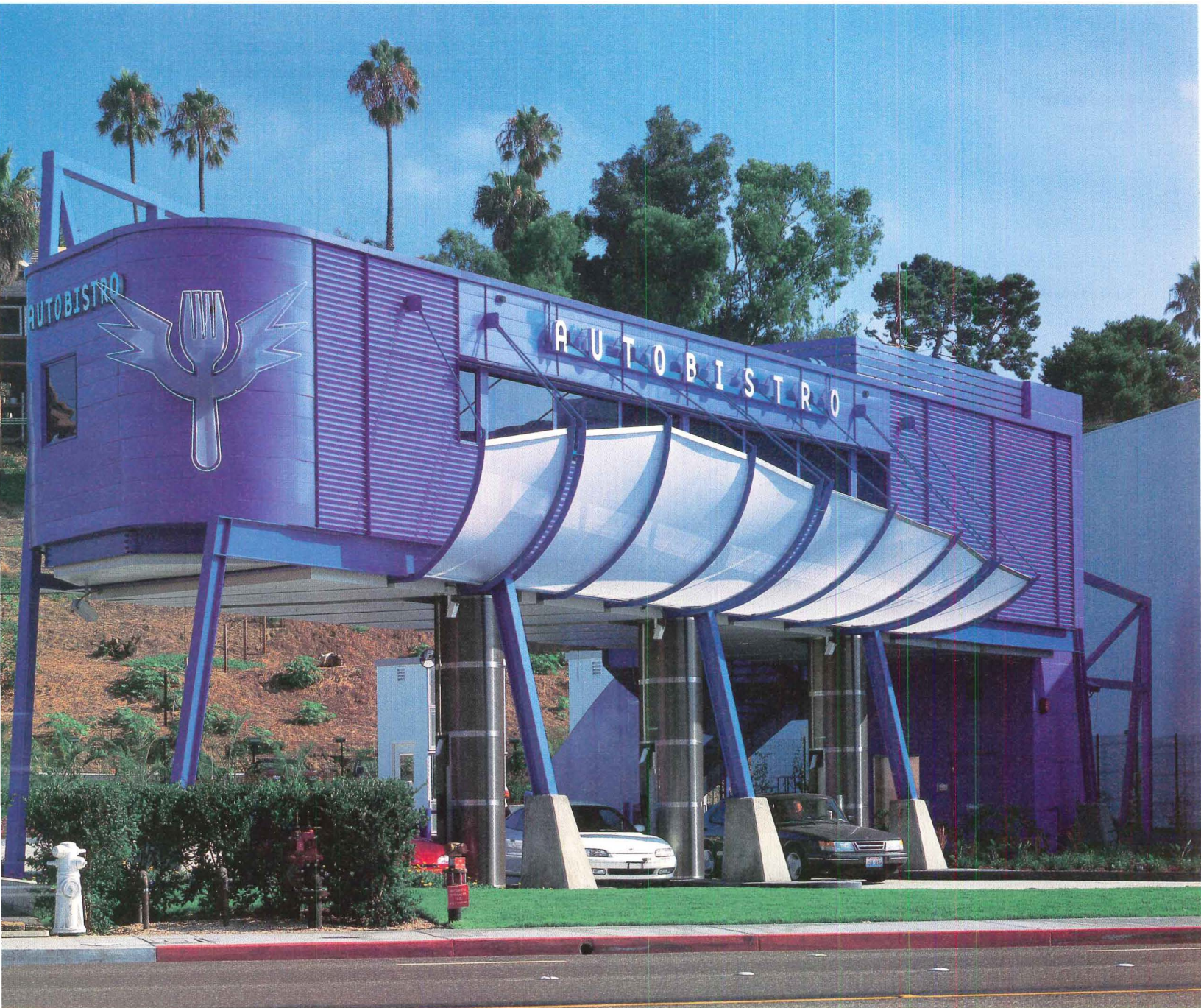
Autobistro's bold colors and sharp, angular forms (above) recall optimistic spirit of early Modernism, according to architect Stanley Boles. Roadside facade sports company's name and winged fork logo. White fabric sail, a gesture to seaside surroundings, partially shades strip windows along kitchen. "Vittleveyors," dumbwaiters that descend through steel-clad tubes, deliver food to drivers parked beneath kitchen.
