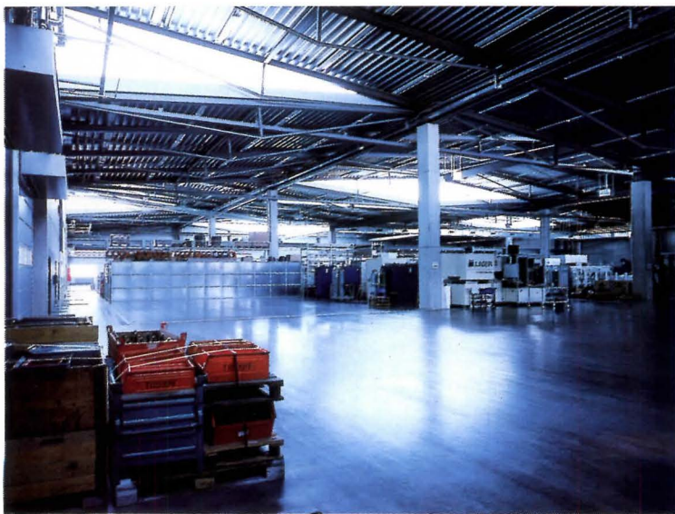
Large metal canopy (top) shelters loading dock that services storage hall at south end of factory. Horizontal bands of zinc clad shedlike structure. Inside storage area (above), gently folding planes of standing-seam aluminum roof create diamond-shaped clerestories that fill vast interiors with daylight. Site plan (facing page) reveals pattern of offset, staggered bays of factory addition, which echoes patchwork of surrounding farms. Tunnel beneath access road connects existing campus to east with new annex. Future expansion will fill open space to west. Autobahn is south of factory.
