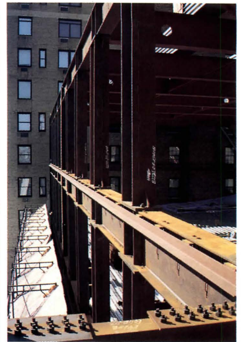
Illustration shows Butler Rogers Baskett's three-story addition (above left) to roof of St. Bernard's School in New York City. Scaffolding with aluminum and translucent panels (above center) protected existing school's top floor from elements when contractors removed roof. Two-story Viereendeel truss system (above right) supports rooftop addition.
