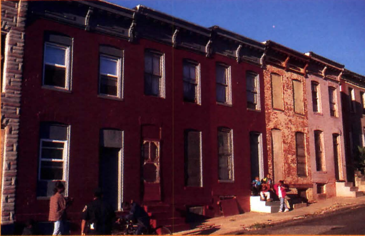
Rowhouses on Llewelyn Street (c. 1885, above) are scheduled for demolition. Buyers revitalized similar structures on Barre Circle (right) under city's 1970s-era Urban Homesteading Program.
