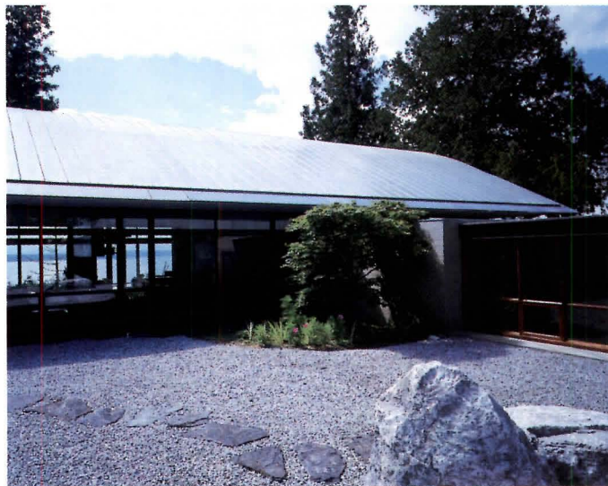
Berthy House (1966, above) in Seattle, Washington, features curved, corrosion-resistant roof of pure zinc.
