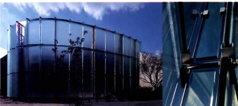
Artist James Carpenter's "Scrim Wall" (above left) encloses open, sun-washed sculpture court that adjoins museum entrance. Steel armature supports individual panes of laminated, patterned glass (above right and detail) that refract sunlight into bright shards of color.
