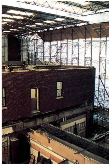
Illustration shows Butler Rogers Baskett's three-story addition (above left) to roof of St. Bernard's School in New York City. Scaffolding with aluminum and translucent panels (above center) protected existing school's top floor from elements when contractors removed roof. Two-story Viereendeel truss system (above right) supports rooftop addition.
