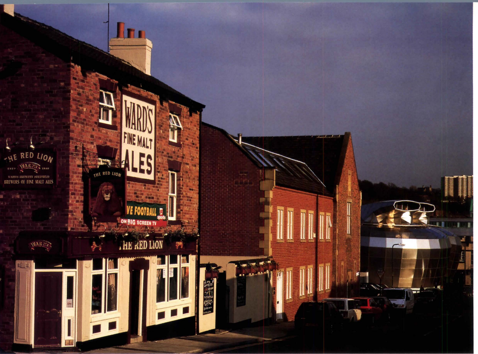
Kettle-shaped, stainless-steel drums of pop music museum (above and facing page, top) peer out from gritty urban landscape of Sheffield's Cultural Industries Quarter. Glass canopy between drums (facing page, bottom left) marks entrance. Stair inside cruciform gallery (facing page, bottom right) connects second-floor exhibits to cafés, classrooms, and gift shop on ground floor.
