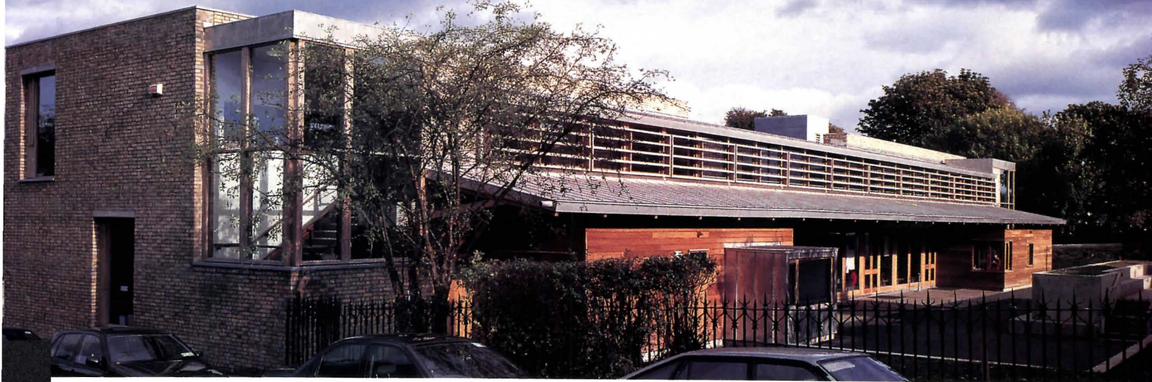
Facing small playground, rear elevation (above) is more open and transparent than street facade. Sloping zinc roof reaches down in welcoming gesture embracing school's occupants. Timber-clad office wing nestles comfortably beneath roof; long veranda provides generous covered play area. Louvered wood screen encloses circulation spine.
