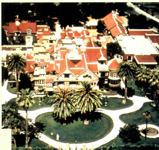
Carpenters worked for 38 years—until owner Sarah Winchester’s death in 1922—on ever-expanding Winchester Mystery House in San Jose, California.
