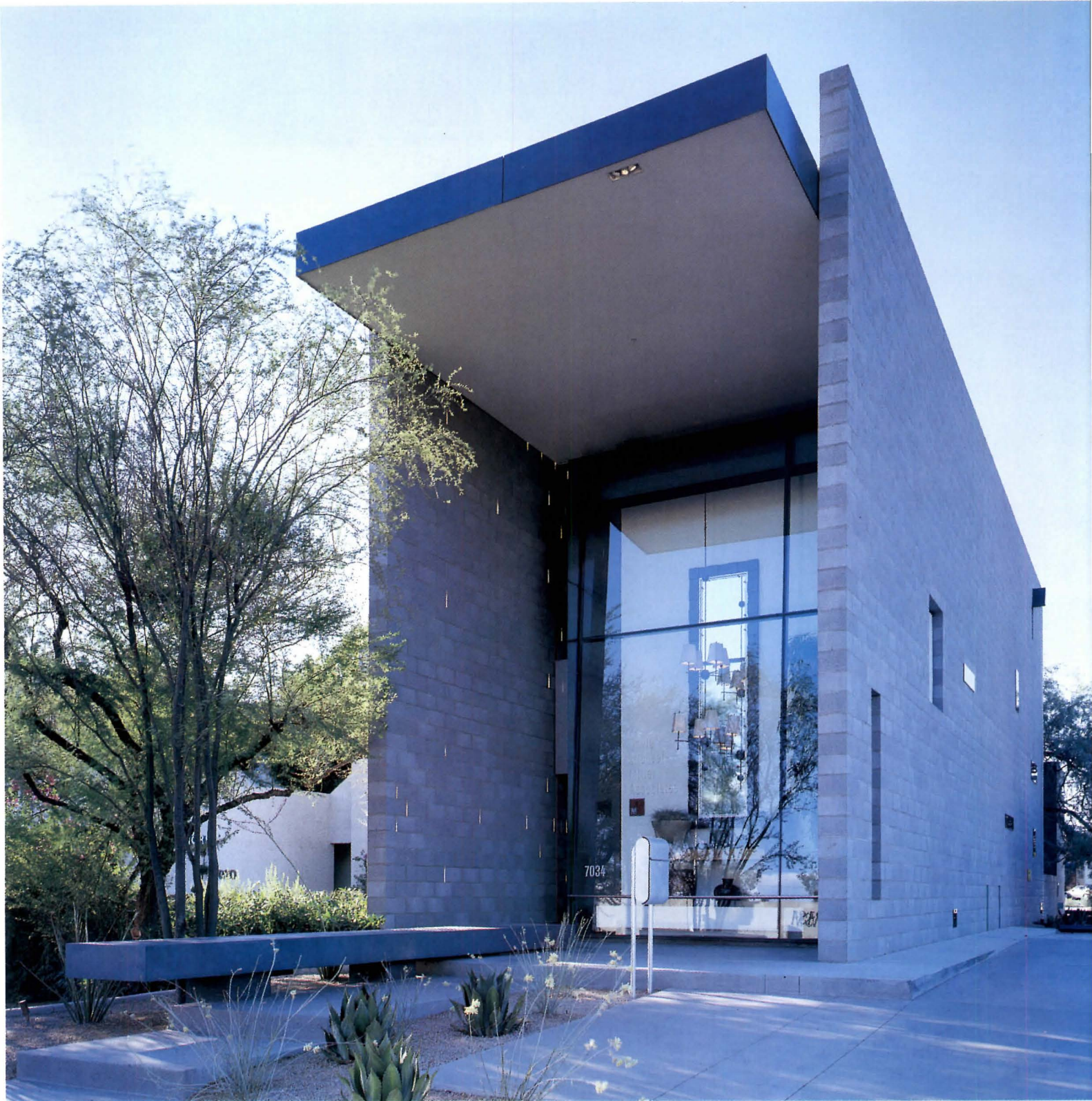
Shaded by overhanging steel canopy, double-height vitrine of entry facade opens onto urbane little plaza (above). Tiny glass strips embedded between blocks of western wall (at left) create luminous streaks. By day, trees cast shadows against hefty concrete block scrim of east elevation (facing page, bottom). At night, light glowing through random pattern of windows (facing page, top) reveals masonry wall's thinness.
