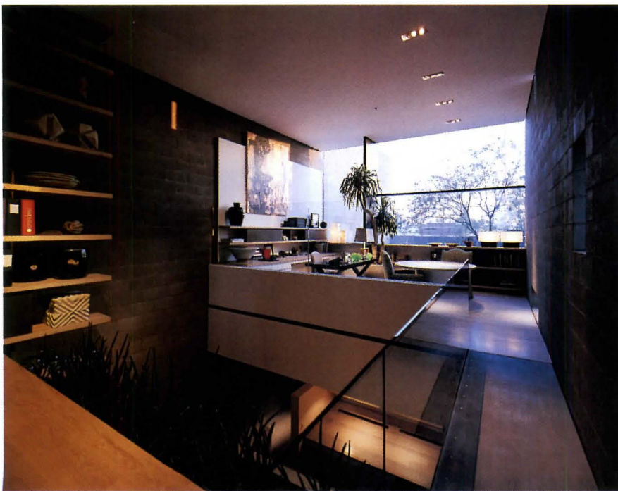
On second floor, cable-stayed steel bridge protected by canted glass railing leads to principal's office at rear. Burnette likens open, airy office to choir loft.
