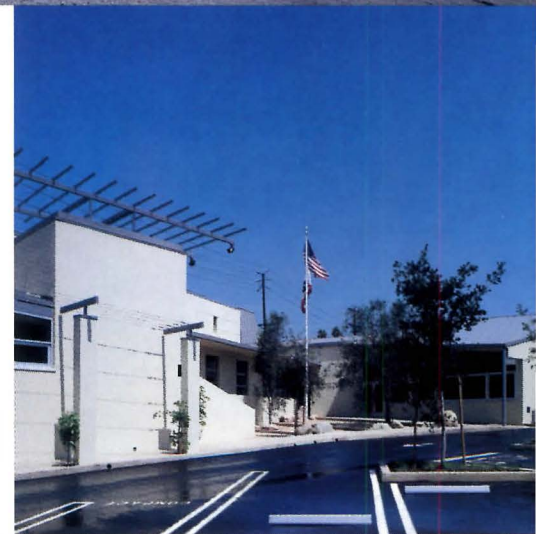
Tilted windows angled into west facade (above) afford corridor parallel to stacks direct view of landmark Griffith Park Observatory on nearby Mount Hollywood. Tubular steel struts form trellis for wisteria above windows. Geometrically relaxed east facade with entry court (below) faces landscaped parking lot.
