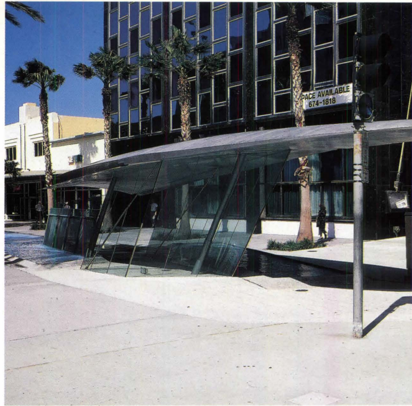
Zapata's pavilion is a contemporary version of the shelters (left top and bottom) built along Lincoln Road during its 1960s heyday by legendary Miami Beach architect Morris Lapidus. The new building's dramatically arced roof (above) cantilevers toward the street through two traffic lights. A portion of the glass enclosure rises from one of the two pools around the pavilion (facing page, right and far right).
