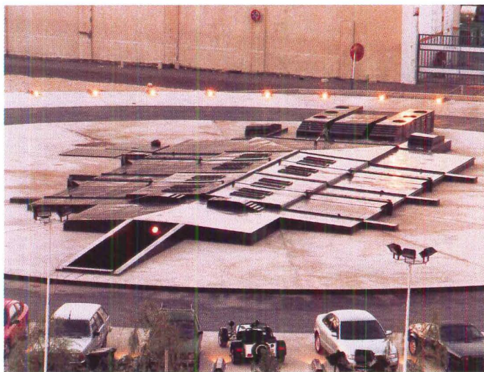
Exposed pistons (above) indicate the roof's retractability; cars park around it in radial formation. The bar appears poised for attack (right) at the edge of dense downtown Beirut, on a site that once served as the city harbor's quarantine station.
