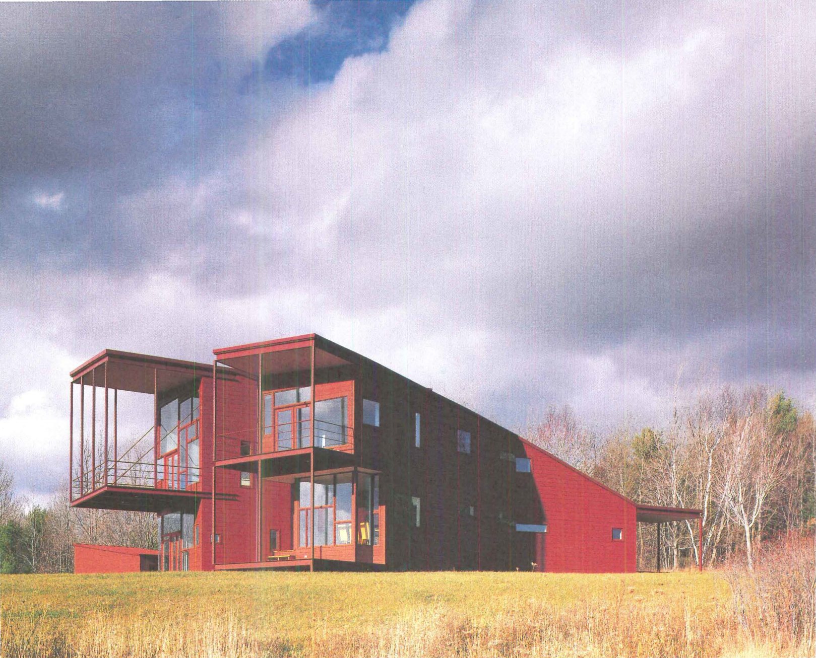
Holl's early sketch of the project (facing page, bottom) and the finished house (above) reveal his clear concept of a split volume. As revealed in sections (facing page, top), Holl located the bedrooms for two generations of family members in separate branches and on separate levels to maximize privacy (below left). On the west-facing ends of the blocks, slender steel members support balconies (facing page, center) facing mountain views. The balconies' horizontal members continue the banding of the painted cedar siding (below center). Seen from the east (below right), the house flares upward and out from its low entry facade.
