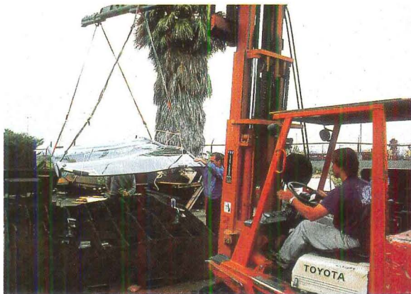
The panels were formed by slumping two sheets of tempered glass over a steel mold. A fiberglass blanket between the glass and the steel (top) prevented the two materials from sticking together in the 1,200-degree oven. Before installation, the panels were loaded with sandbags (center) to check deflection and verify live loads. Finished panels were carefully lifted (above) and loaded on a flatbed truck for delivery to the site. Each panel is dramatically different from any other one. Computer renderings (right) reveal the range of undulations in panels 1 through 5.
