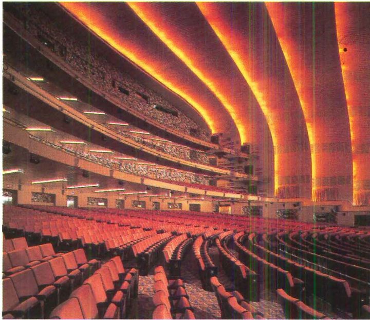
A newly woven, 112-foot-wide gold curtain hangs from 13 motorized cables concealed behind the restored proscenium's overlapping arches (facing page). All 5,910 original seats in the 450,000-square-foot auditorium were replaced (below). The ceiling was resurfaced with coats of metallic speckled paint (above).
