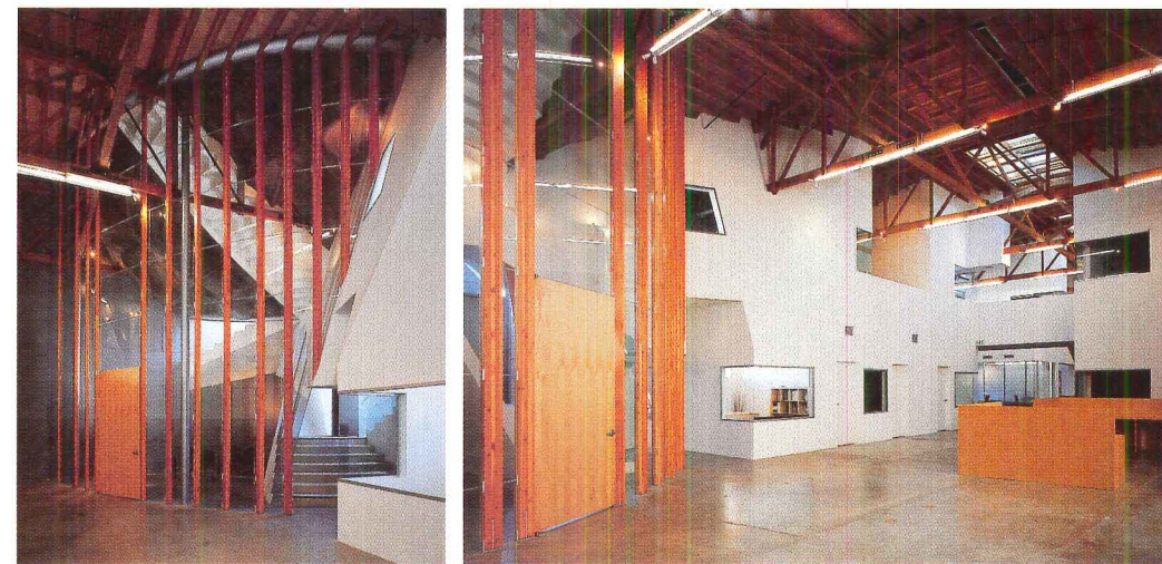
A conference room (far left) sits immediately beneath the Umbrella canopy, at one end of an open work floor (left). Lapped sheets of glass in a wood frame enclose the conference room (above left); the underside of the concrete stairs and gunnite roof form its ceiling.
