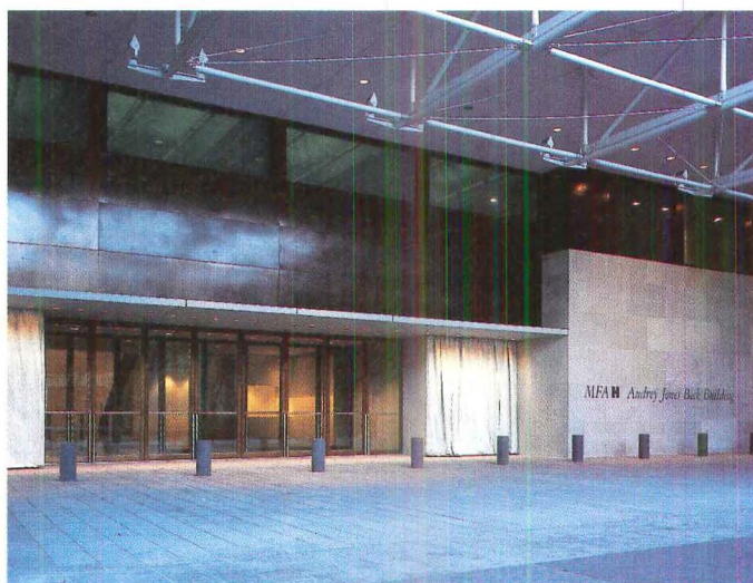
The canopied north entrance (facing page) bridges another entrance below grade. A waterfall (top left) mirrors exterior stairs that lead to the basement entrance. The granite-clad drive-through (top right) on the west facade also serves as an arcade sheltering the main entrance. Moneo surrounded the front door (above) with bronze panels and a curtainlike sculpture by Joseph Havel.
