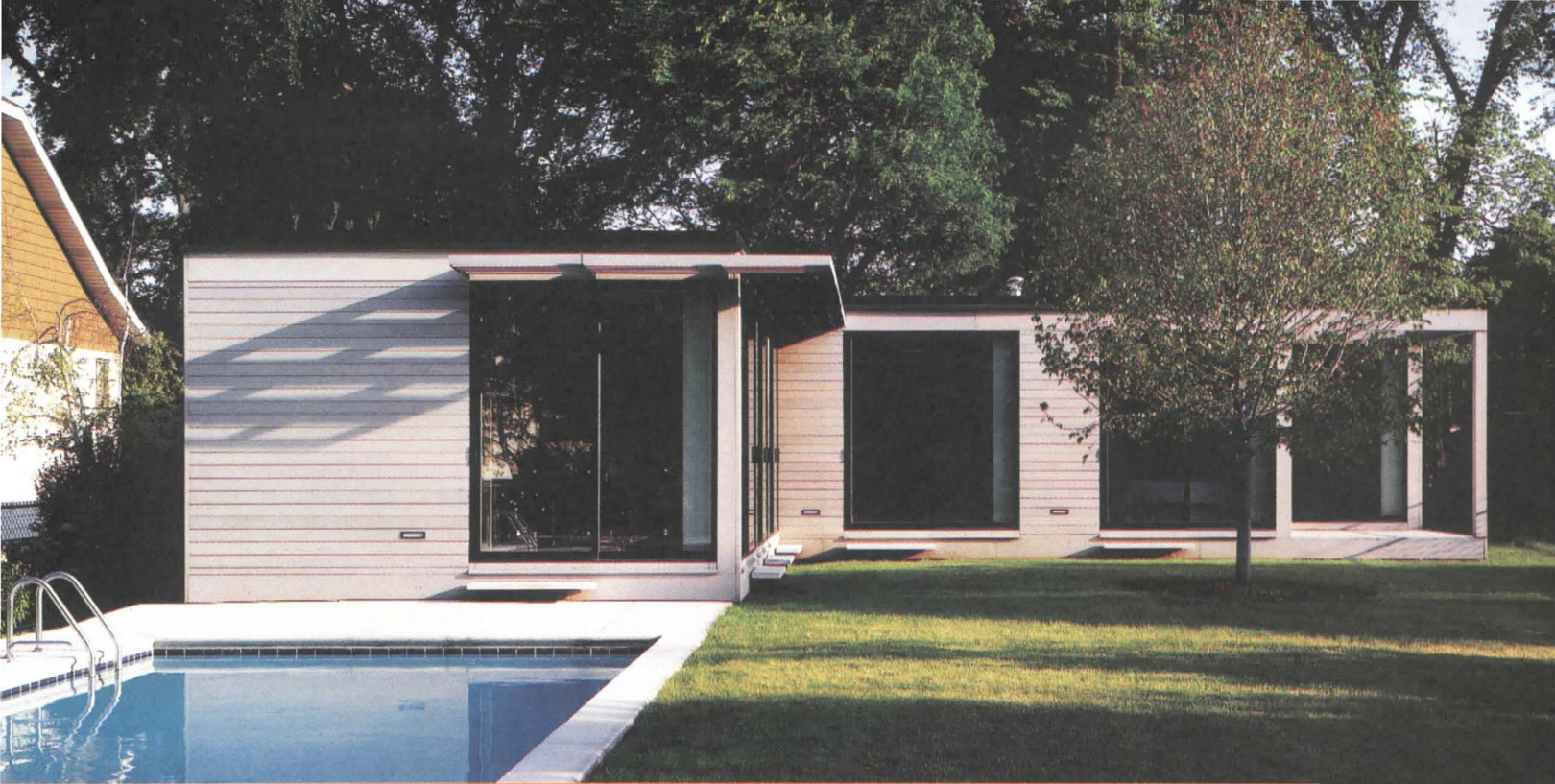
The T-shaped plan of the Wangler house creates discrete public and private zones on a modest Chicago-area lot (above, and previous pages). A 2-by-6 wood frame construction clad in clear cedar siding is affixed to lath strips and attached to the walls to create an insulating air space (below right). The living room is clad in maple plywood, as are the kitchen cabinets (below and bottom left).
