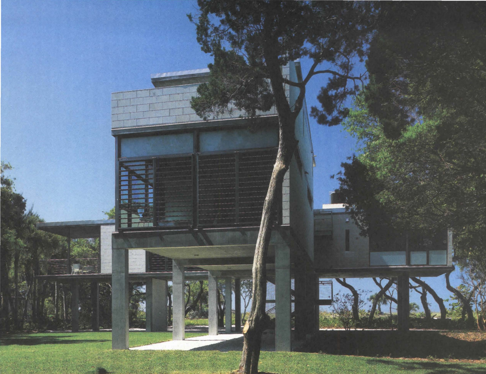
Toshiko Mori's addition to a central Florida estate, anchored by an original Paul Rudolph house, stands a full floor above the ground plane among a grove of live oak trees (previous pages). The concrete frame and off-the-ground stance meet Florida hurricane standards while also providing shady retreats from the sultry climate. Windows are protected by powder-coated stainless-steel louvers (facing page and above). Mori's design had to conform generally with the size and placement of a house that previously occupied the site.
