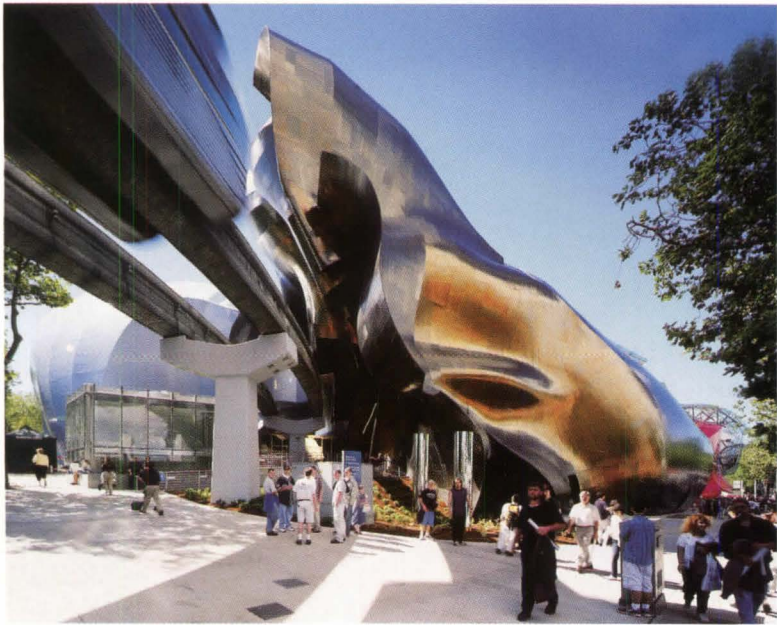
The monorail penetrates the south end of EMP (right) through a tunnel (above); its elevated track separates the main body of the museum from the theater, which is sheathed in powder-blue painted-aluminum shingles. The north end of the building (top) houses the restaurant.
