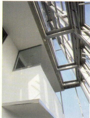
The dramatically sloped façades of Coop Himmelblau's SEG apartment tower in Vienna (facing page) serve as part of a simple, but effective, passive climate-control system. One façade, fitted with computer-controlled louvers, encloses a winter garden (above center). In other apartments, balconies are fitted with windows that can be opened manually (top left and above left).
